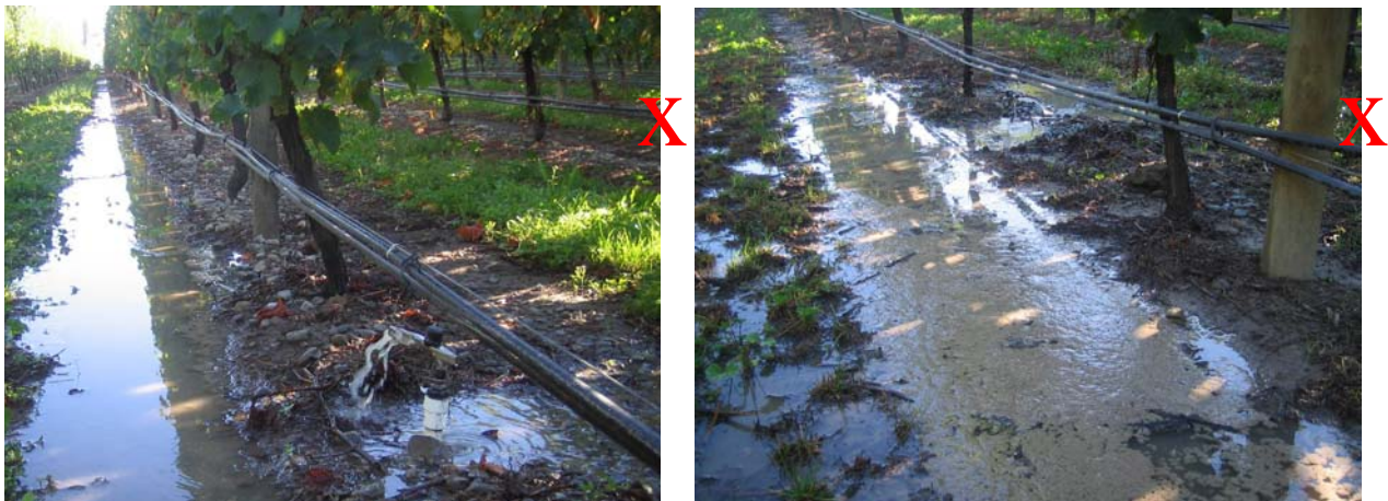
Overloading of Wastewater to Land
