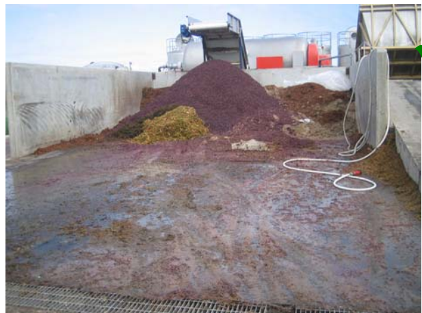
Grape Marc Stored on Concrete Bunded Pad with Leachate Collection
