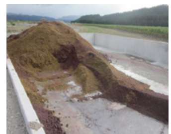
Sealed storage area with leachate collection
