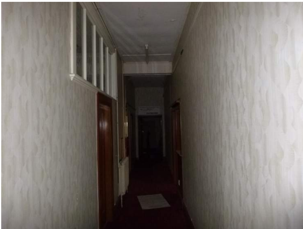
Photo 16: Loadbearing corridors at lower level
