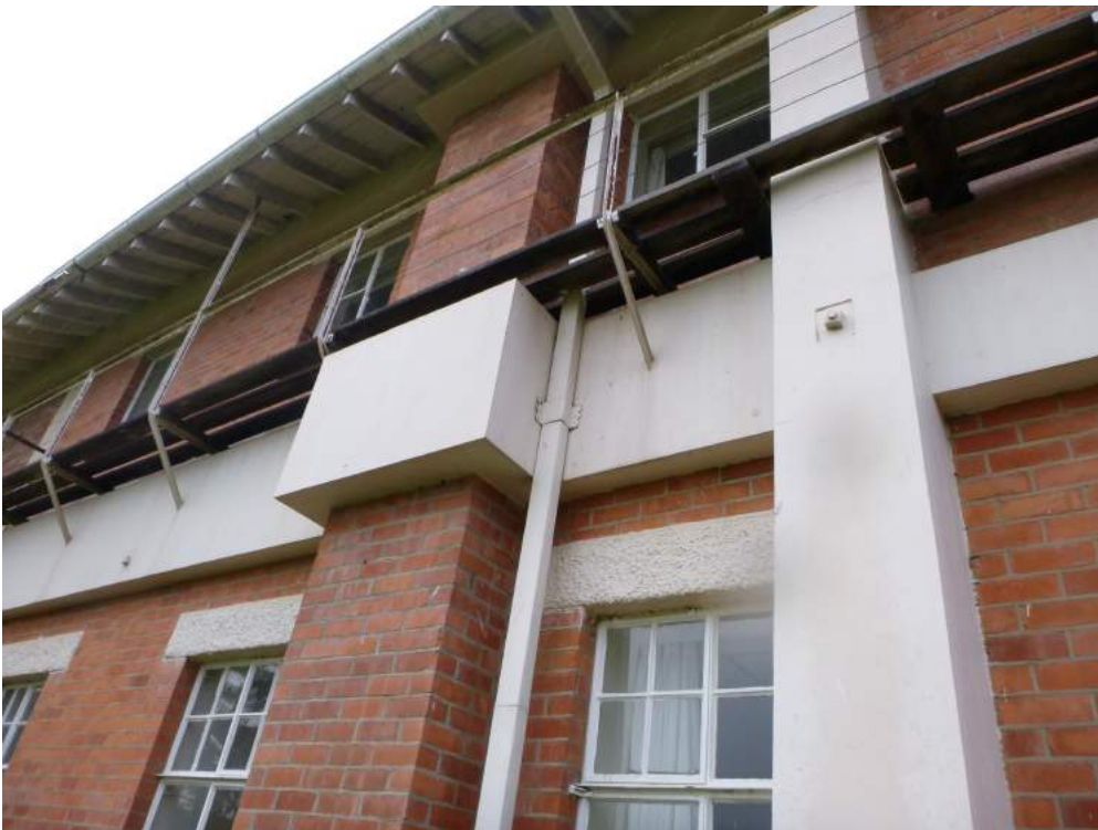
Photo 14: Buttressing and bond beams to original building
