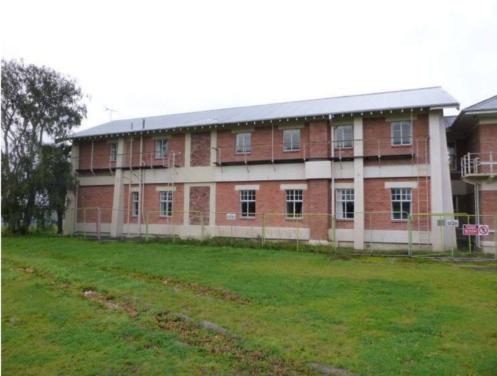
Photo 4: West Elevation – North wing
