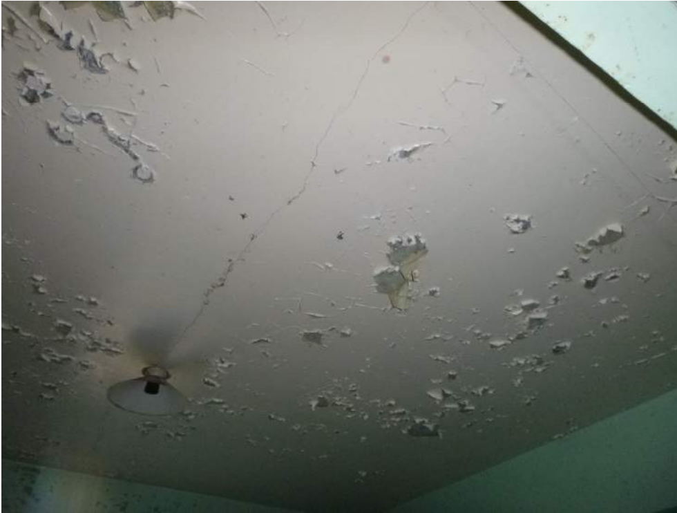
Photo 23: Roof slab over south end of kitchen
