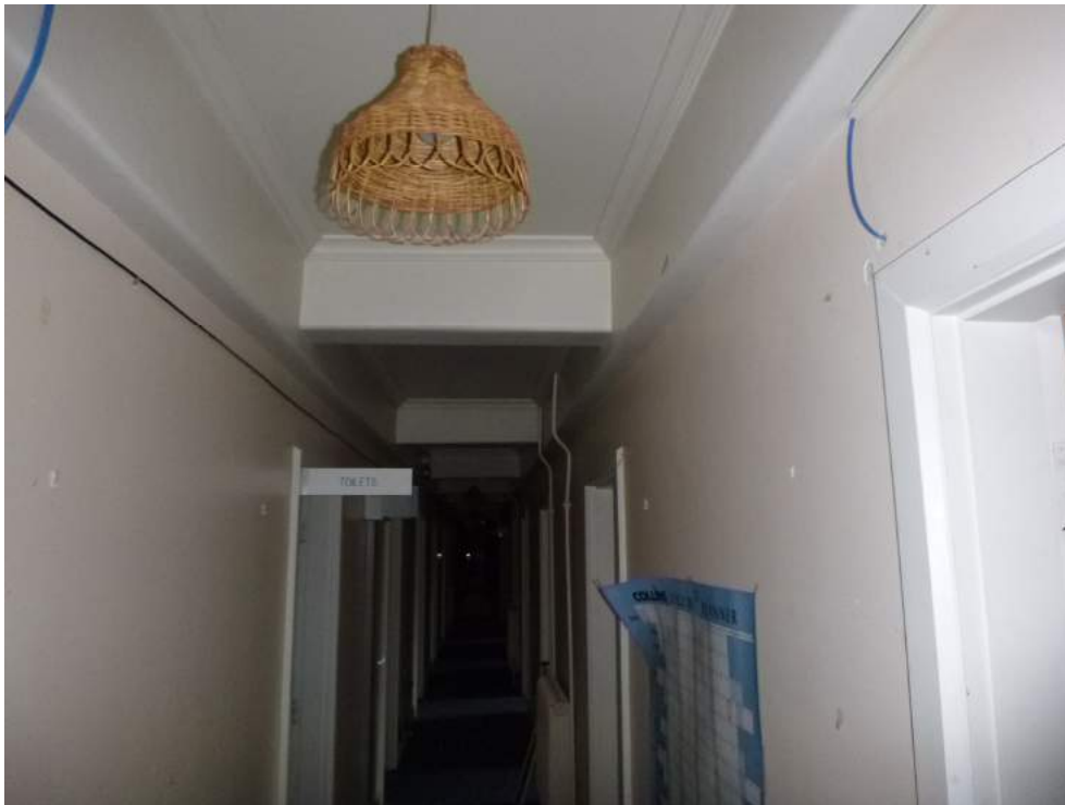
Photo 29: Bond beams over corridors in south-west extension
