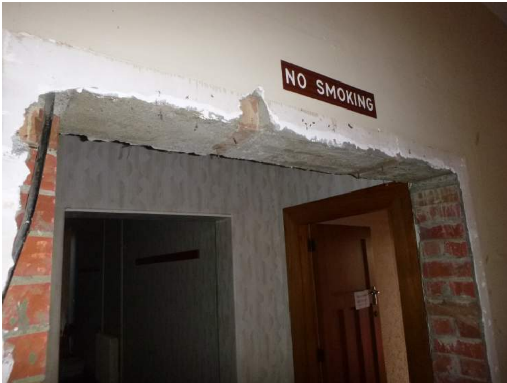
Photo 17: Opening in corridor walls – loadbearing brick
