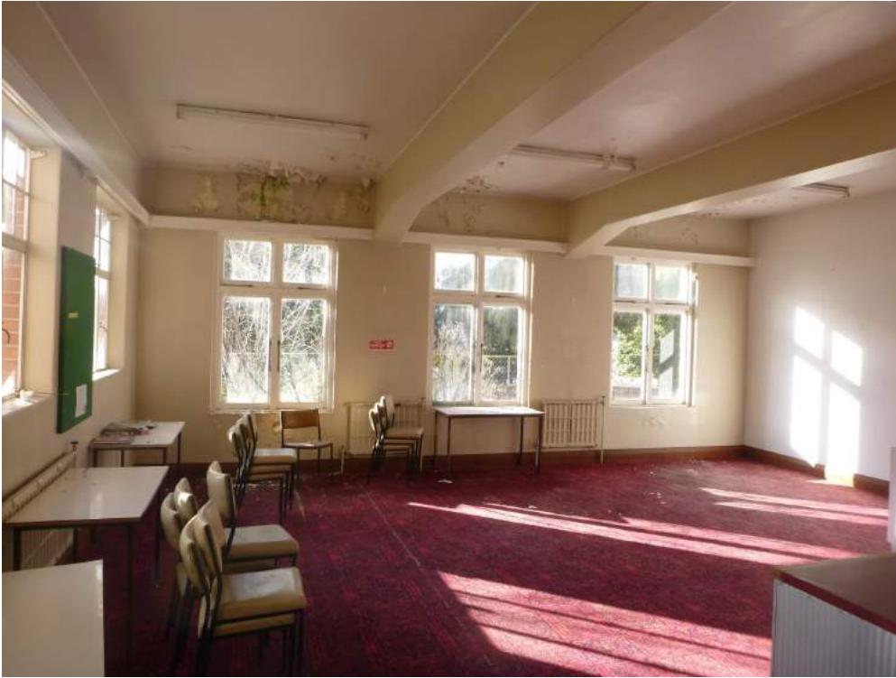
Photo 21: Concrete beams over east side of building – single storey
