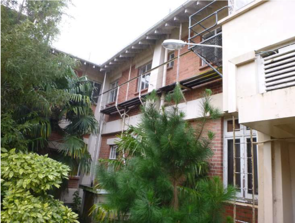
Photo 9: Courtyard West elevation
