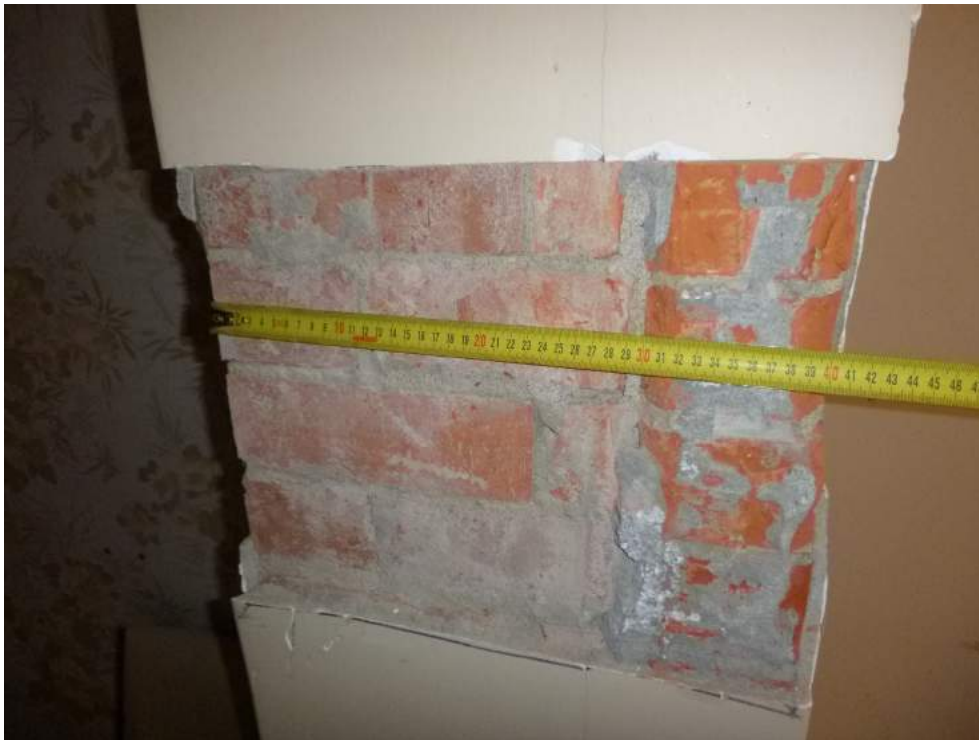
Photo 19: Exterior brick walls of 2-storey building at kitchen
