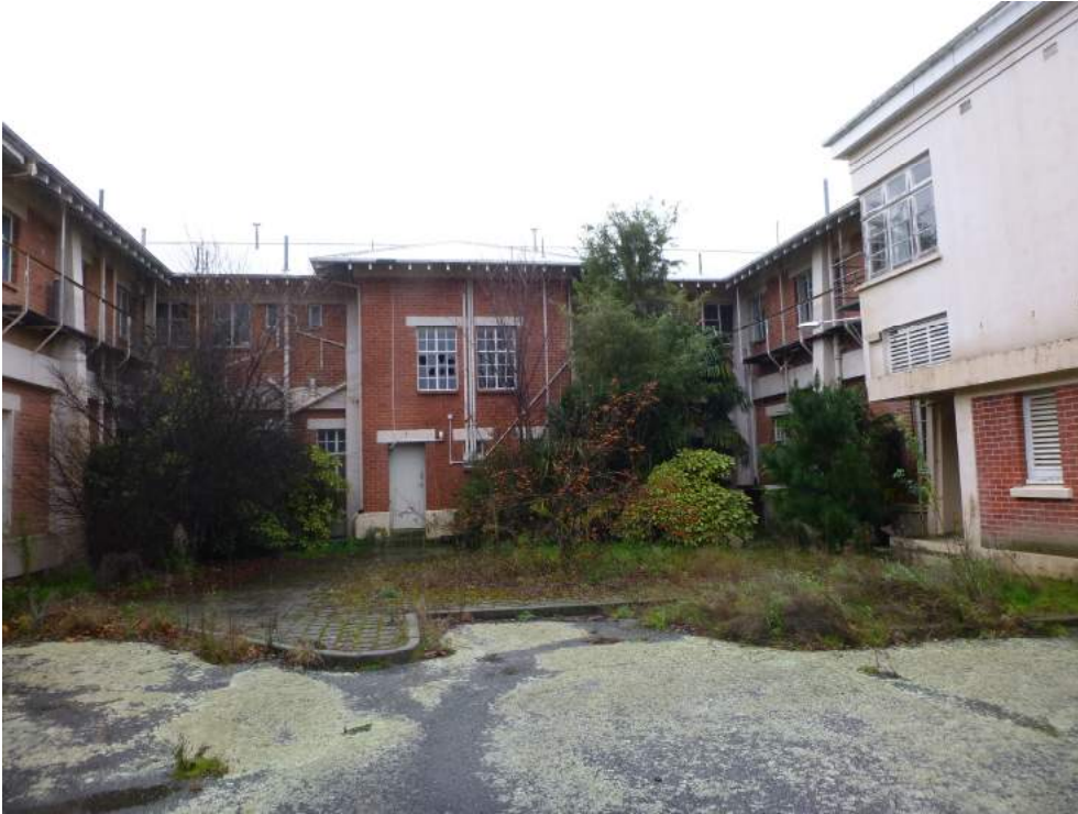
Photo 7: Courtyard South elevation
