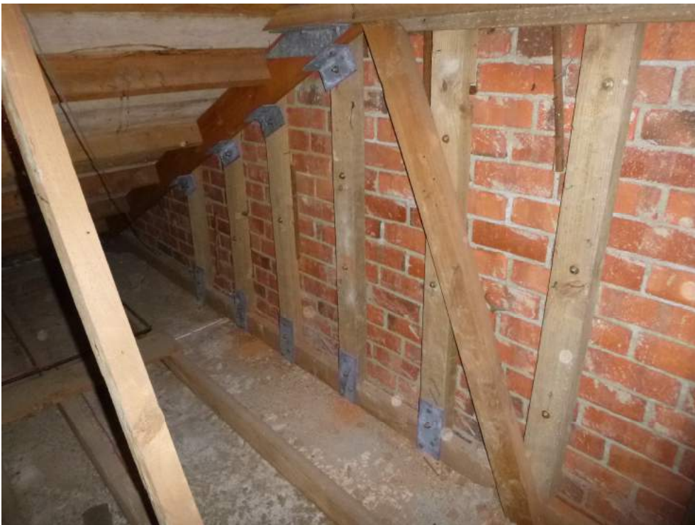
Photo 28: Connection brackets at brick gable wall
