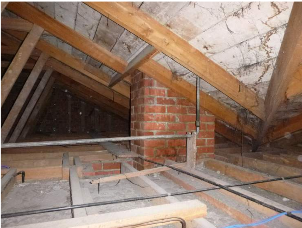
Photo 26: Timber roof framing, timber sarking, brick chimneys
