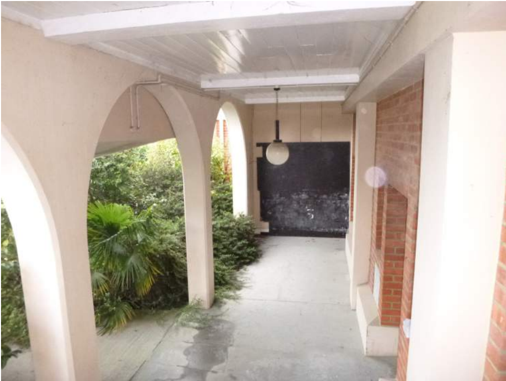
Photo 13: Verandah at north entry area
