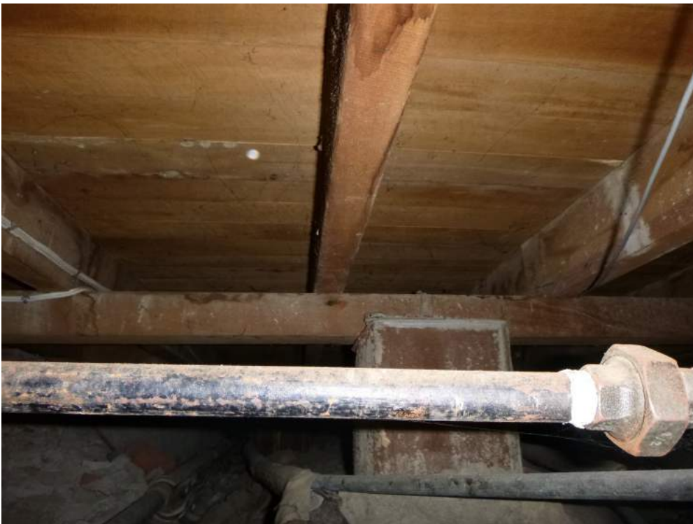
Photo 24: Timber subfloor on concrete piles
