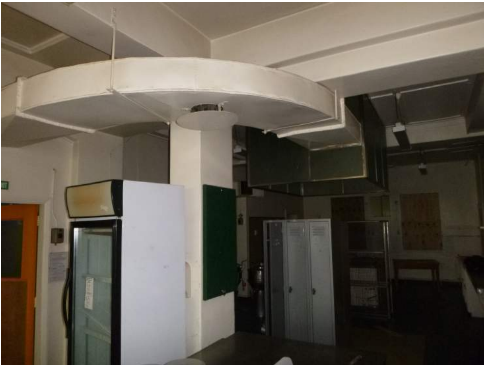
Photo 22: Concrete beams and columns over kitchen
