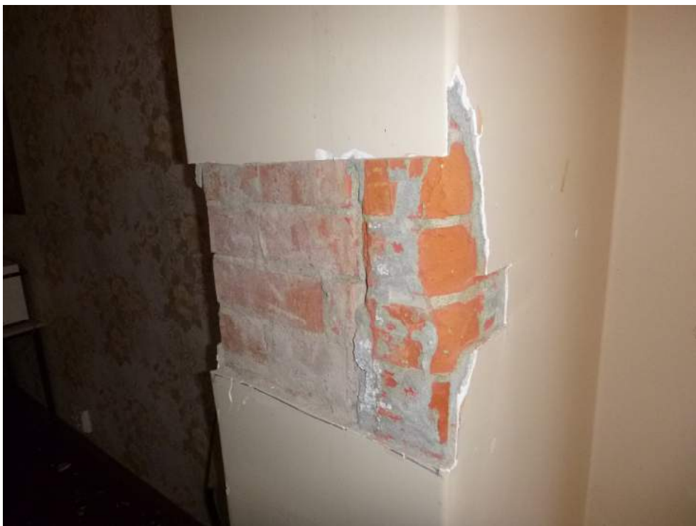
Photo 20: Exterior brick walls at kitchen
