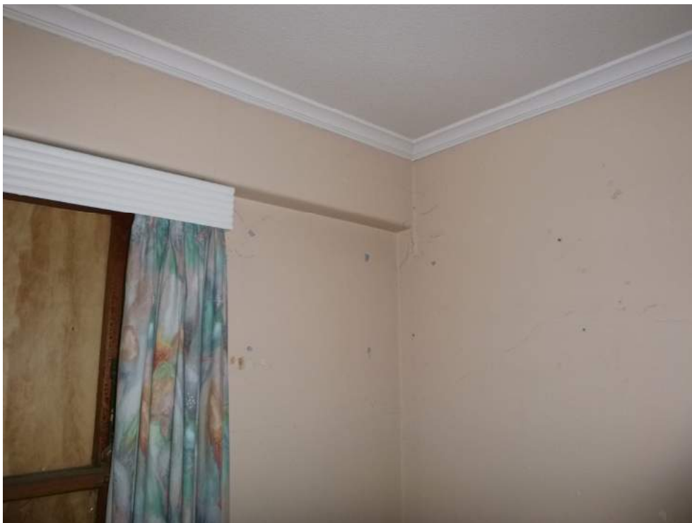
Photo 30: Bond beams over exterior wall in south-west extension
