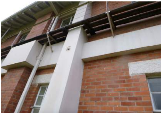
Concrete buttresses and bond beams added to exterior of building
