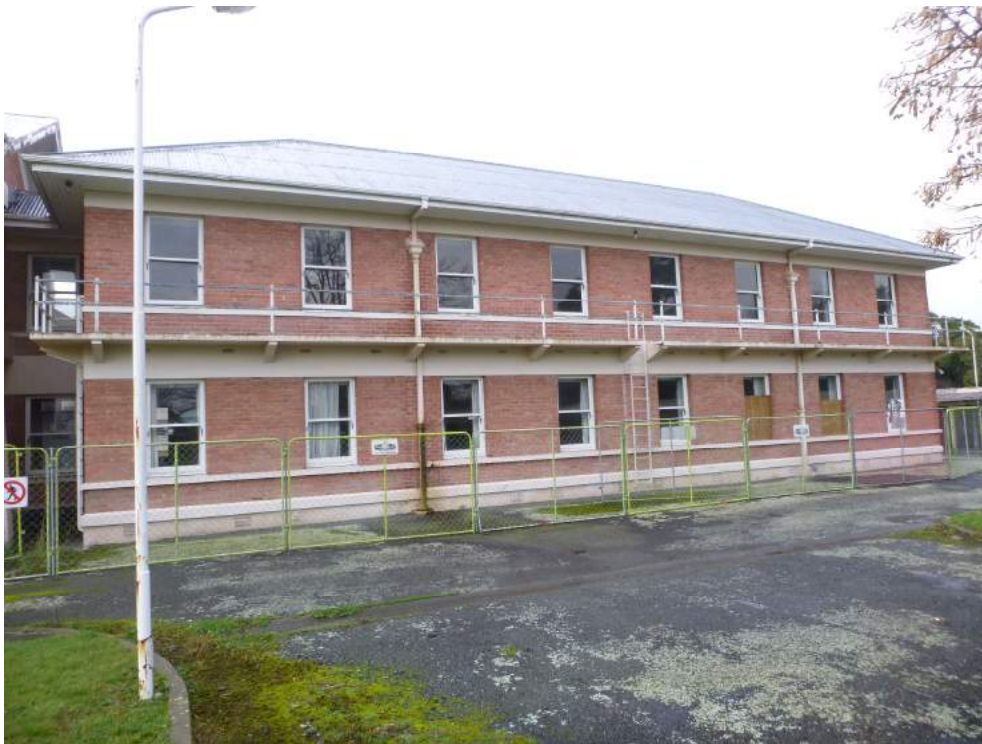
Photo 5: West Elevation – South wing
