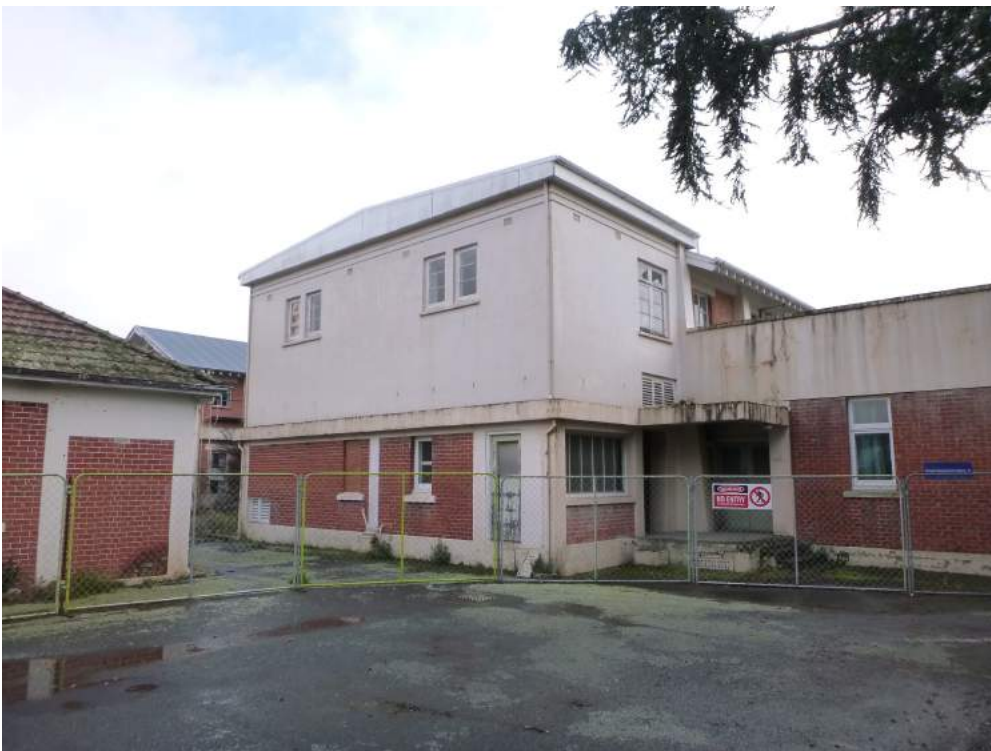
Photo 10: South elevation of East wing
