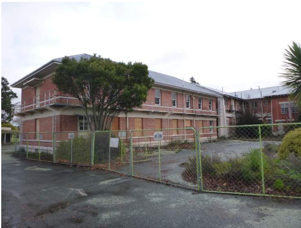
Photo 6: Courtyard elevation – West wing
