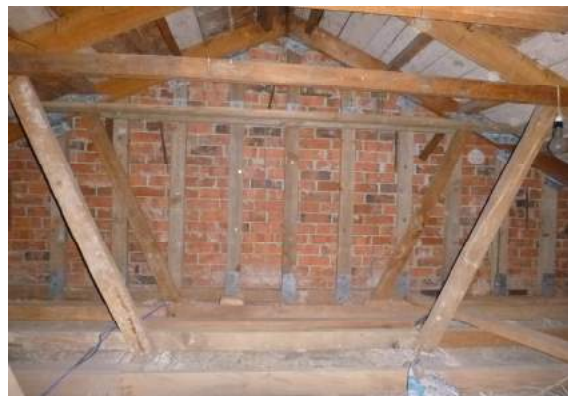
Strengthening to Gable Walls
