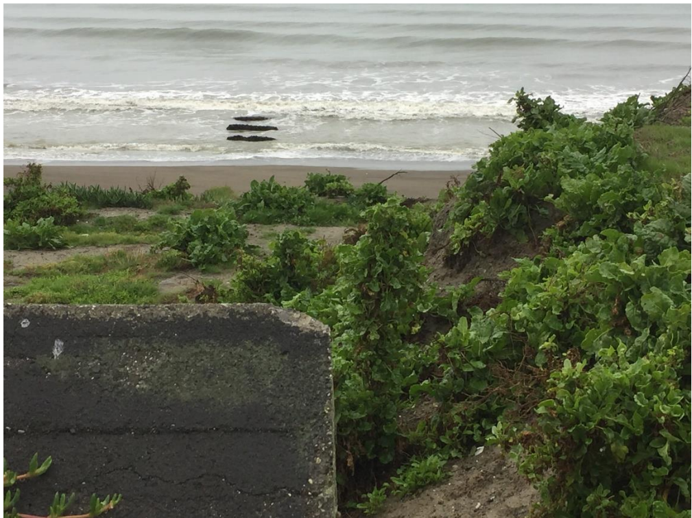
Photograph 2: The old intake pipeline.
