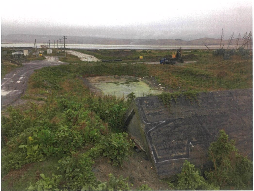
Photograph 3: The settling pond in the area marked as Indicative River Bed Polygon.
