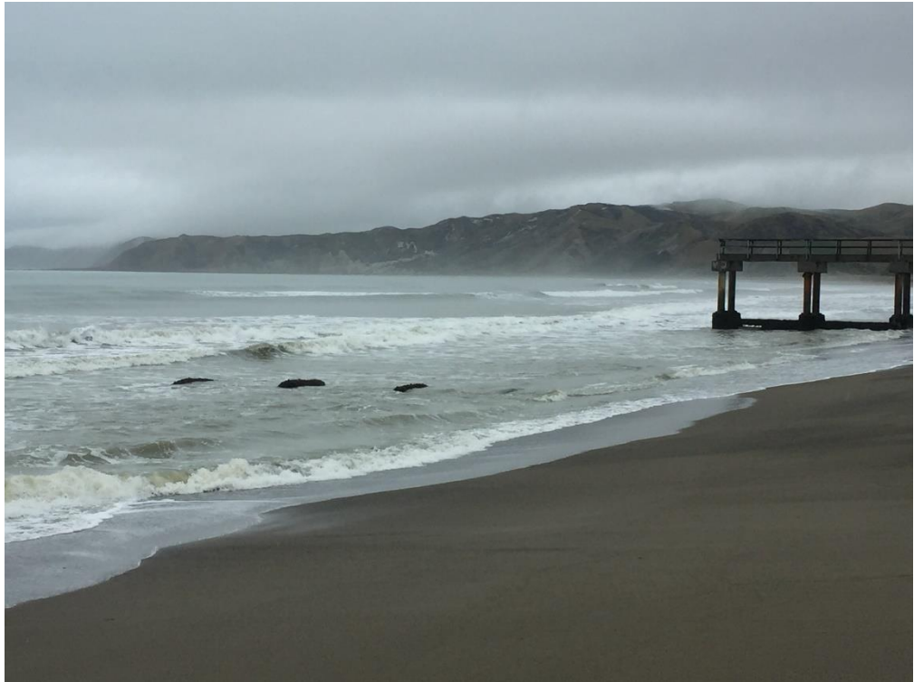
Photograph 1: Part of the old intake pipe is visible (left). The old intake pipe extends seaward approximately the same distance as the current intake pipeline (right).
