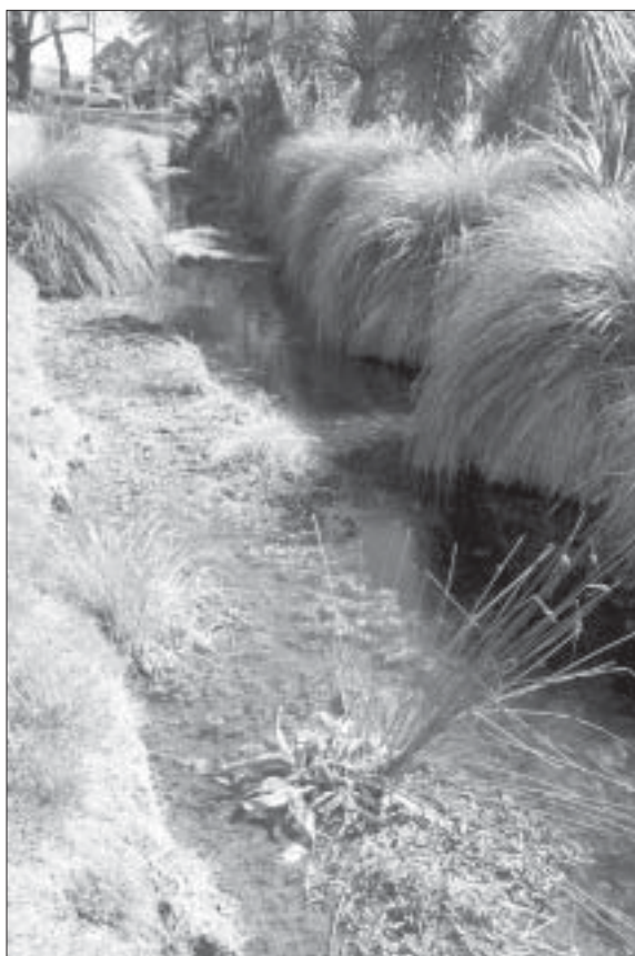
Figure 7. Aquatic macrophytes have been selectively removed to create a meandering low-flow channel, with retention of some in-stream habitat.
