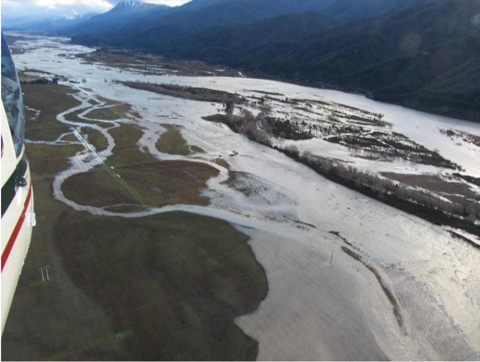
Photograph 1: Site Visit 15 July 2012 – aerial view of vineyard damage
