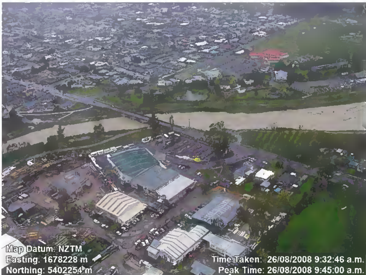
Photo 7: Flood in Taylor during August 2008 flood event
