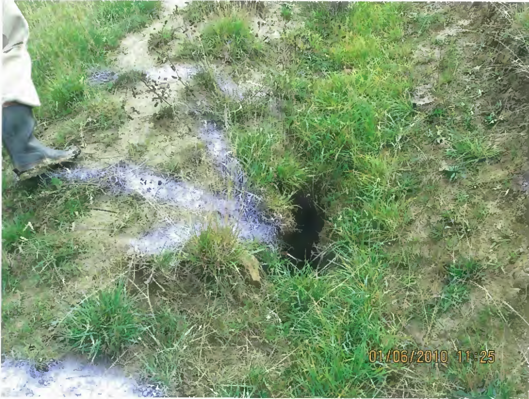
Self-developed hole from cut-off channel down into tunnel gully under-runner
