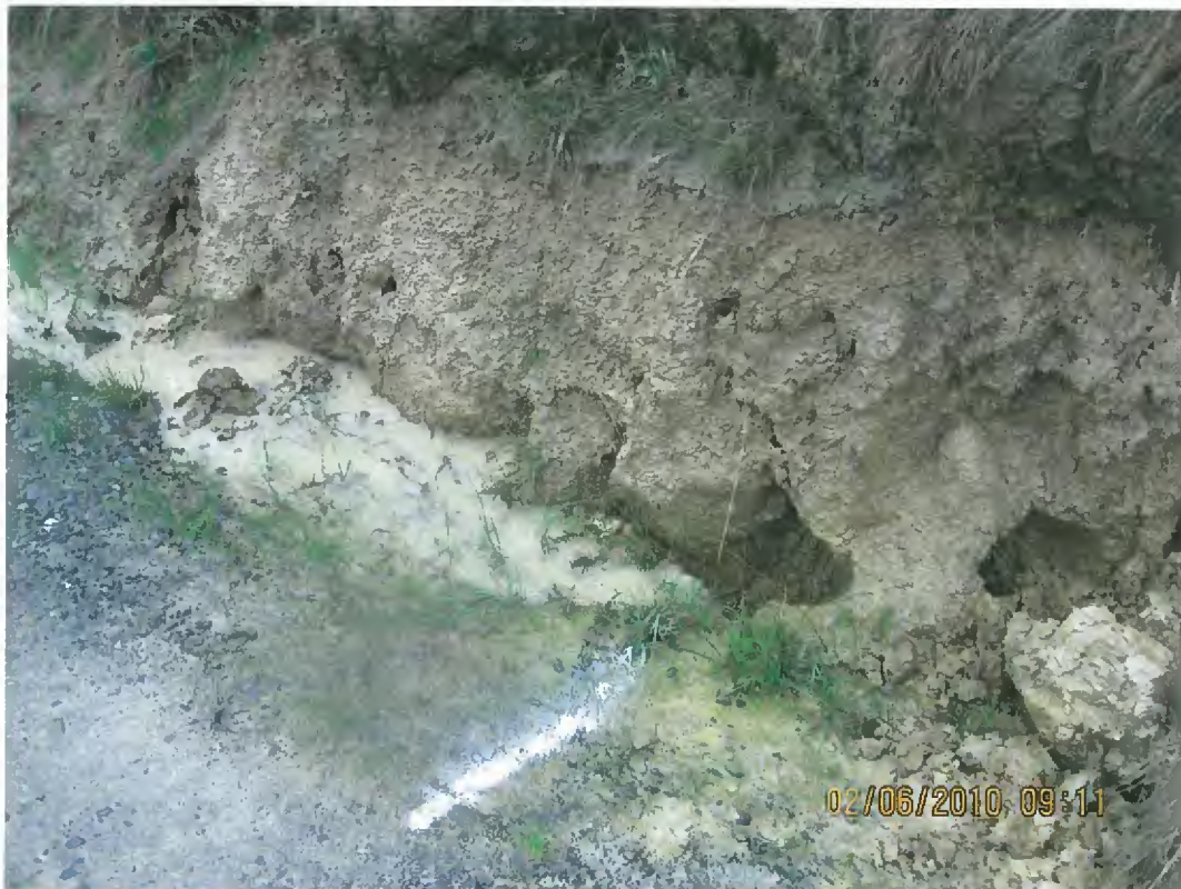
Detail of water disappearing into under-runner
