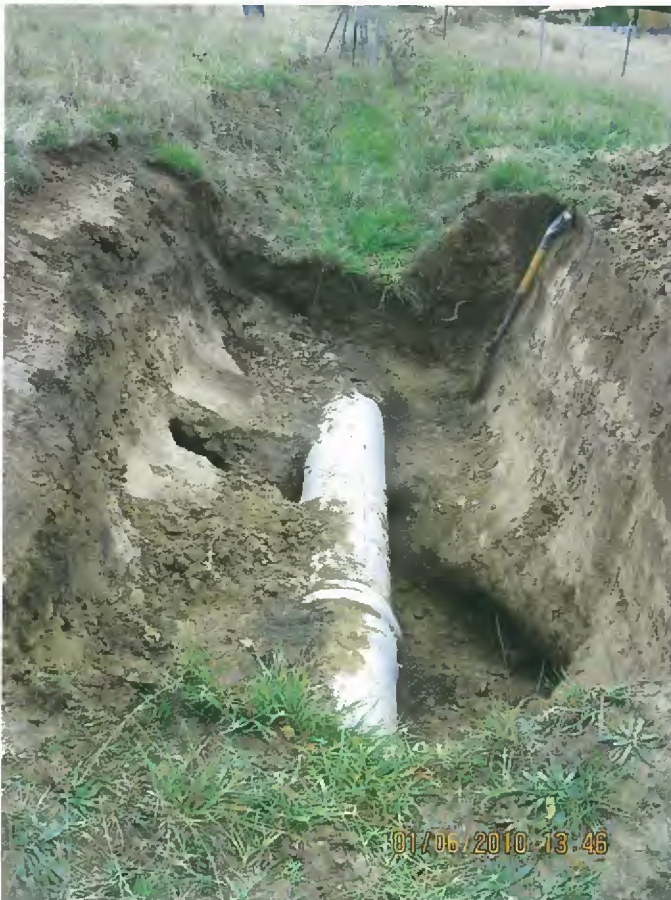
Self-developed hole from cut-off channel down into tunnel gully under-runner
