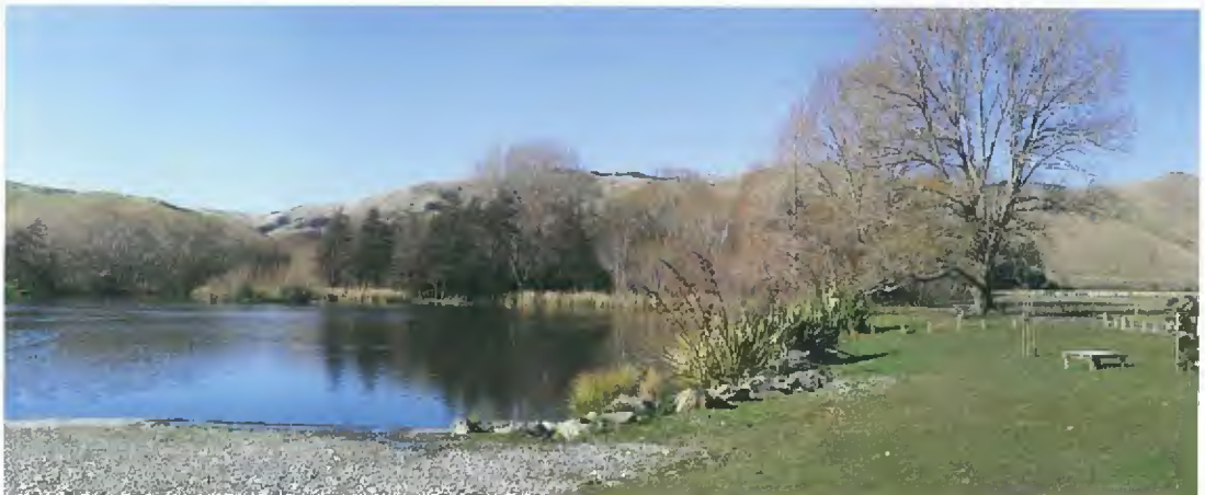
Plate 3: The Taylor Dam.
