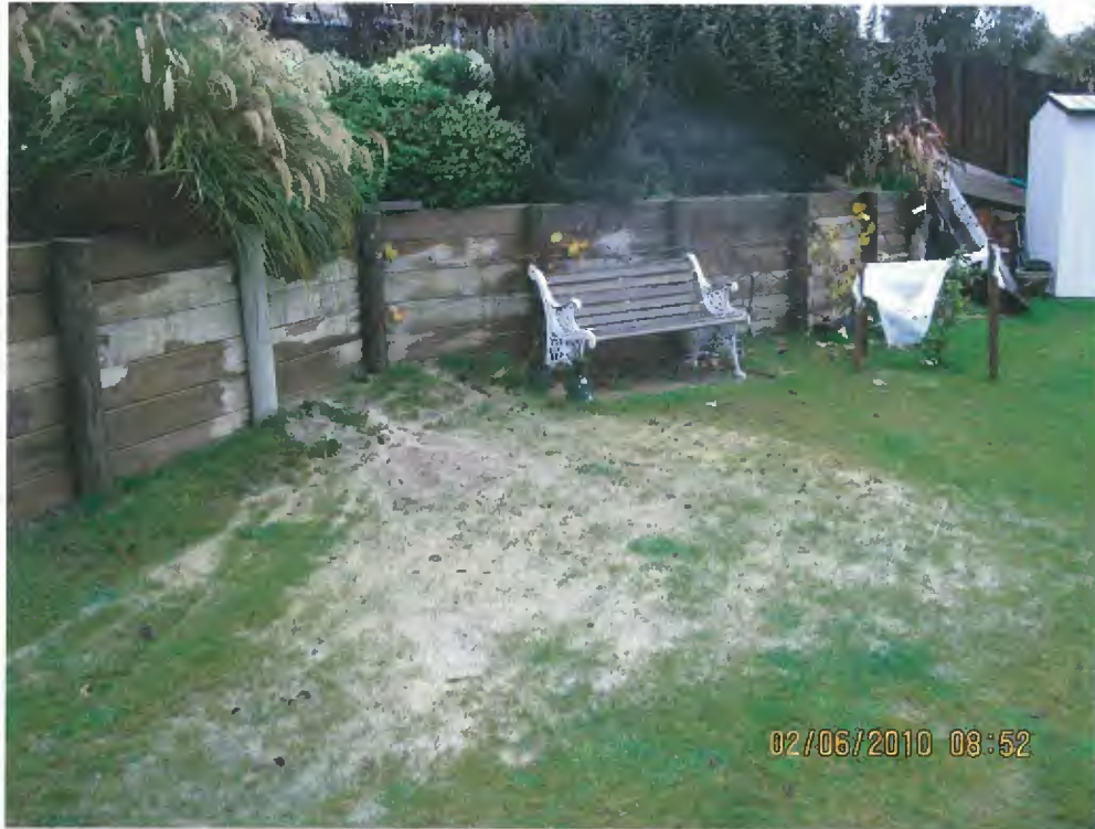
Silt deposited on Reed's lawn from dirty water pushing out under retaining wall.
