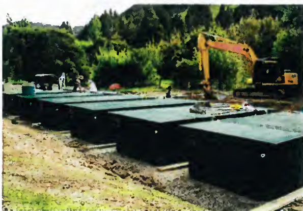
Figure 4: AdvanTex® pod installation - in this case an AX600 rtPBR.
