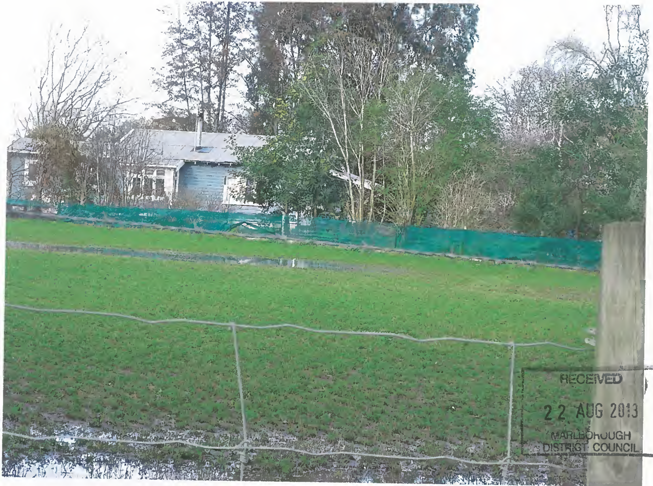
BATTY'S ROAD - 2 houses on lot "family flat" Rural 3 (older house obscured by trees to right)
