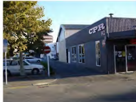
ABOVE FIG. 5-22: Poor quality pavement and insufficient width of the footpath in Wynen Street.
