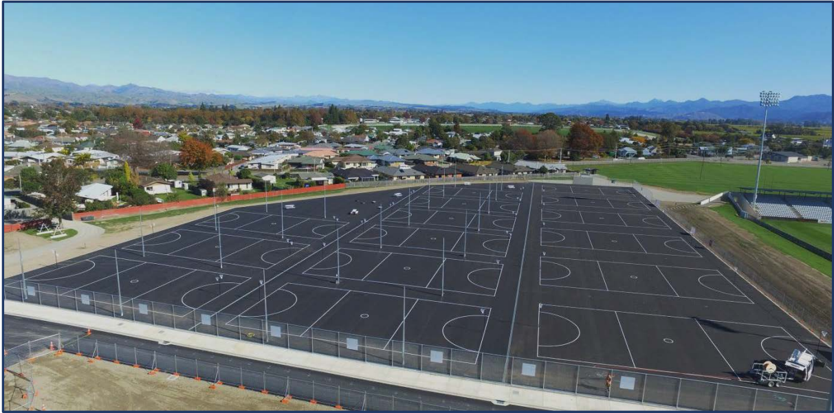
Lansdowne Park netball courts, Blenheim (pre-construction of hub building)
