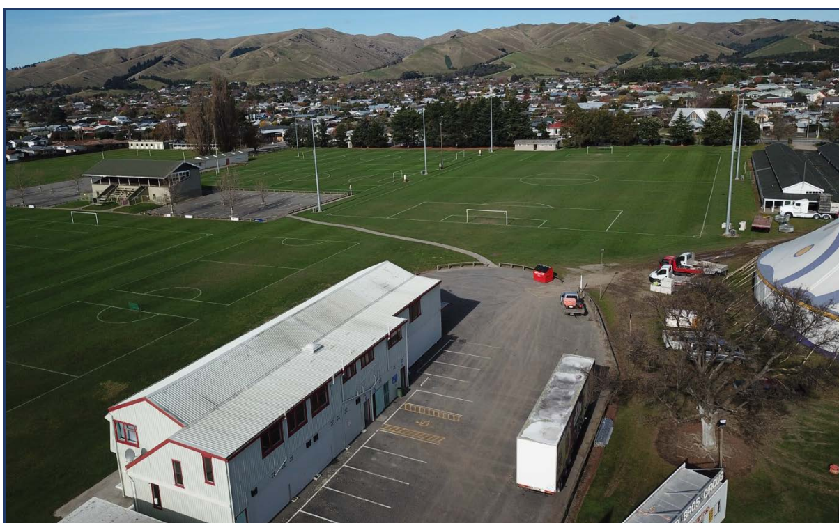
A & P Park, Blenheim (pre demolition of grandstand)
