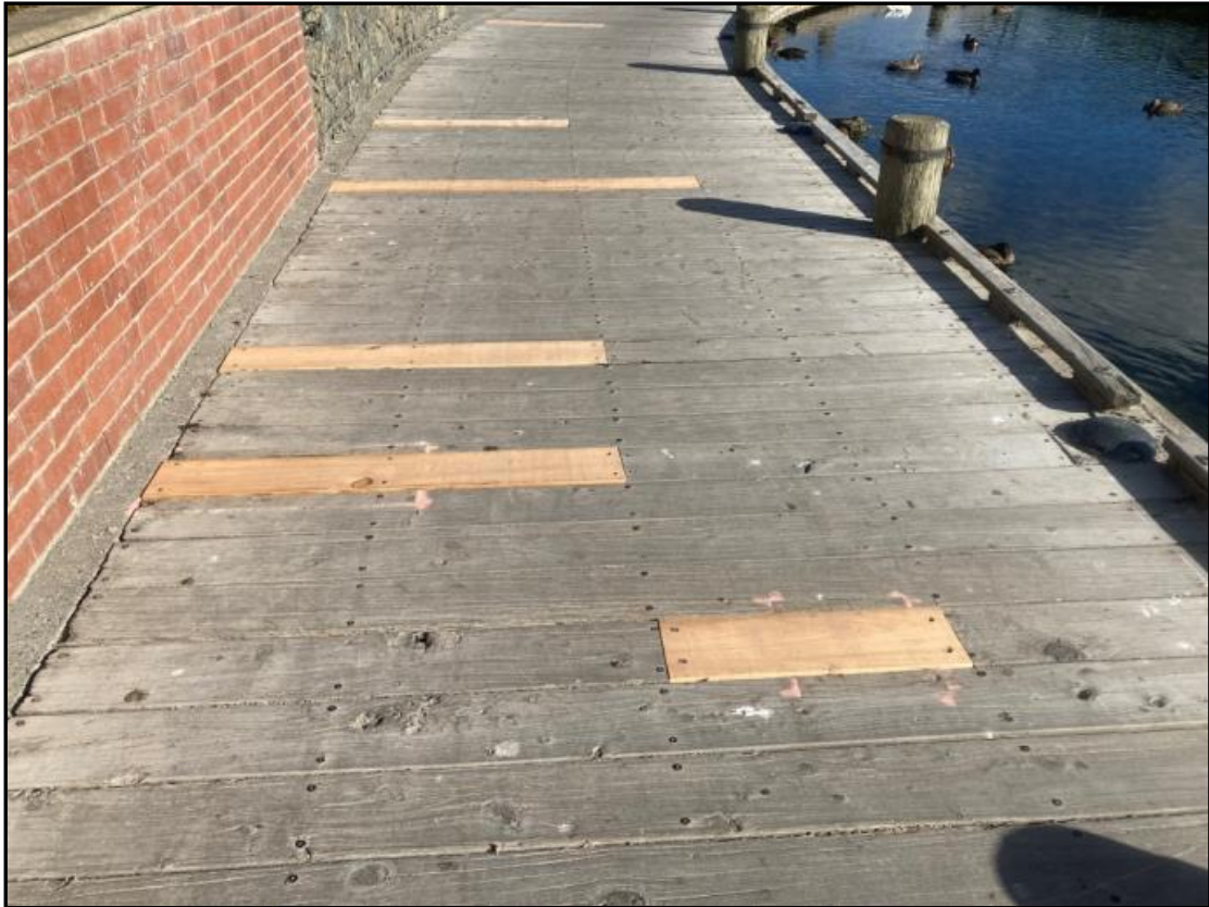
Replaced boards section of pathway
