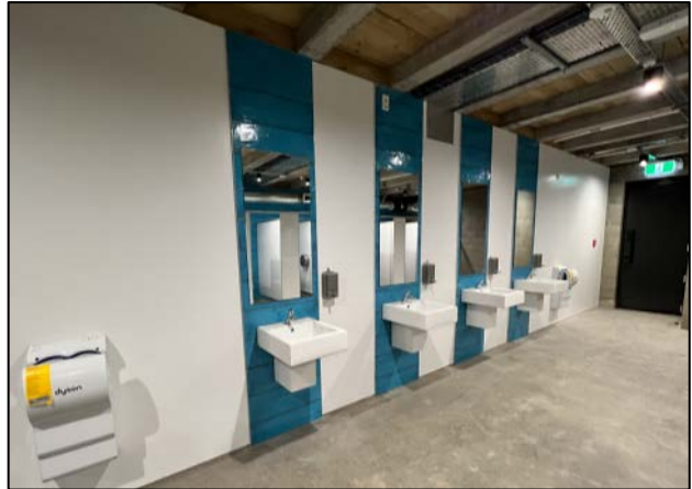
Fig 10 – Lansdowne Hub, Completed women's toilets, ground floor
