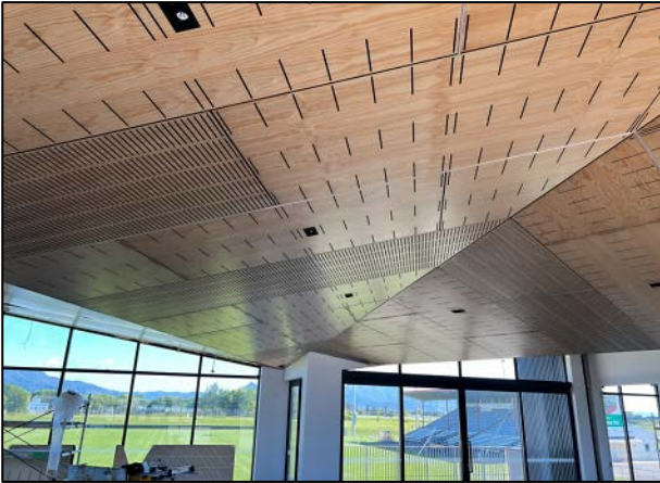
Fig 9 – Lansdowne Hub, completed ceiling, first floor
