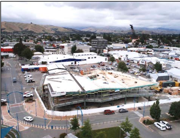
Fig 11 – MLAG, roof progress, Nov 2021
