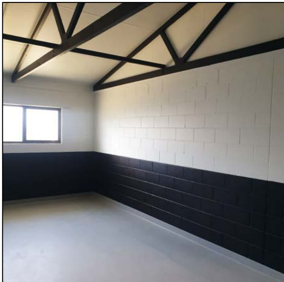
Fig 5 – Moutere Rugby Changing Rooms, new changing room 3
