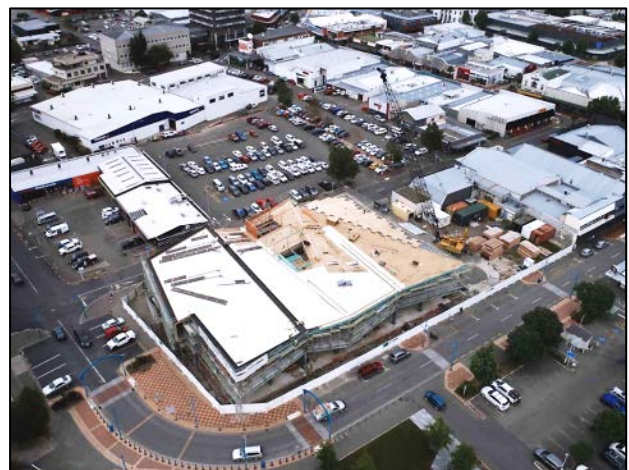
Fig 12 – MLAG, roof progress, Nov 2021
