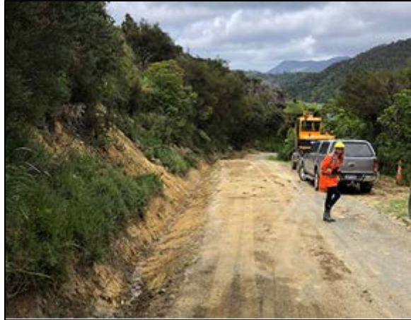
Approximately 5000m 3 of material has been removed
