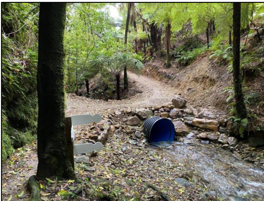
New culvert and track crossing
