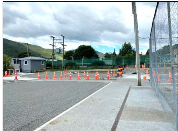
Fig 2 – Neil St Upgrade, new exposed aggregate footpath and vehicle crossing progress
