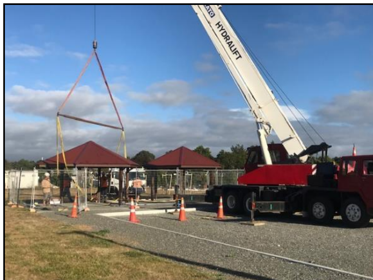
Shelters being craned into place at Omaka Cemetery
