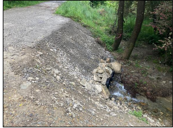
Culvert replacement on Top Valley Road.
