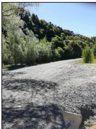
Photo 2 – Running course with large particles migrated to the top due to dry weather conditions.
