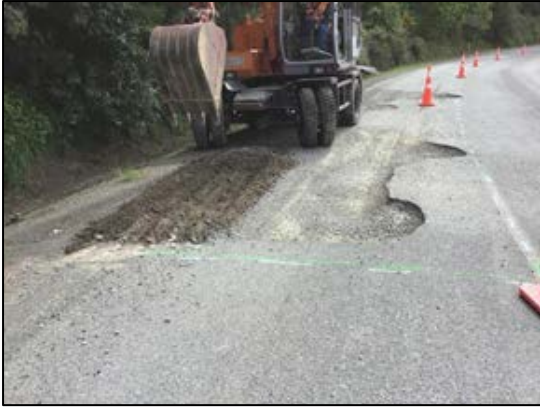
Road repairs: removing damaged seal and replacing with new mix.
