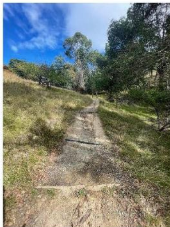
Eroded trail surface on Gentle Annie walking trail. Drainage and resurfacing required; this will also deter riders from using the walking track.
