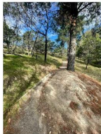
Eroded trail surface on Gentle Annie walking trail. Drainage and resurfacing required; this will also deter riders from using the walking track.
