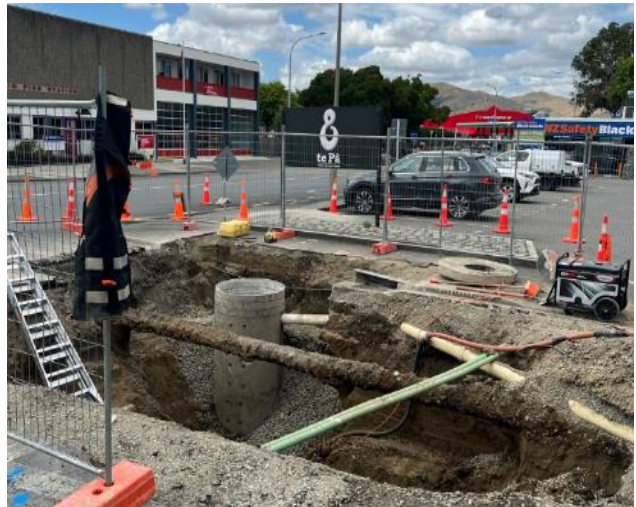
Fig 8 – Storm water upgrade, Blenheim Streetscape
