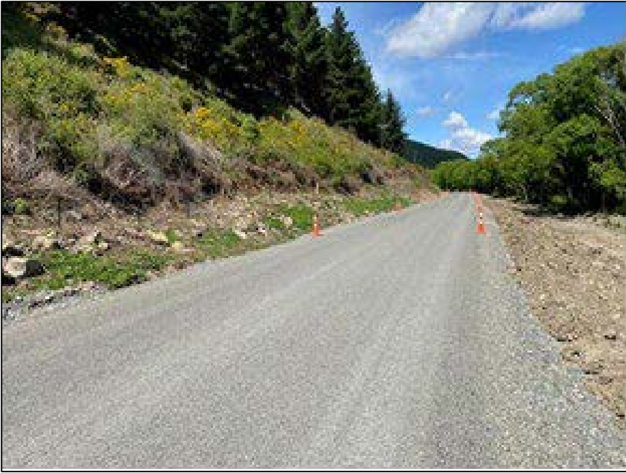
The Waihopai Road Realignment project.
