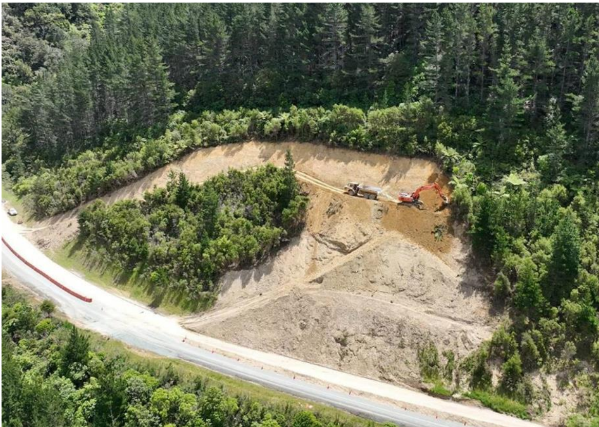
Figure 3: - works being undertaken during SH6 road closure
