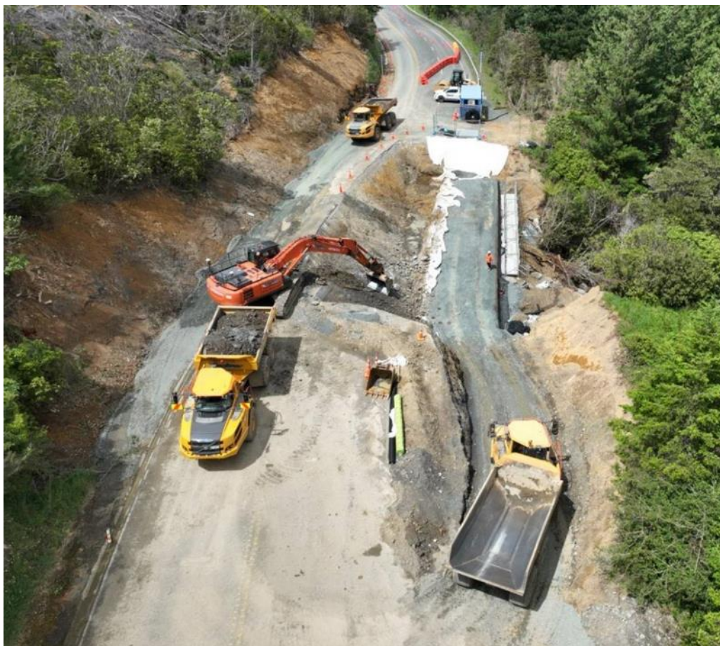
Figure 1: - works being undertaken during SH6 road closure
