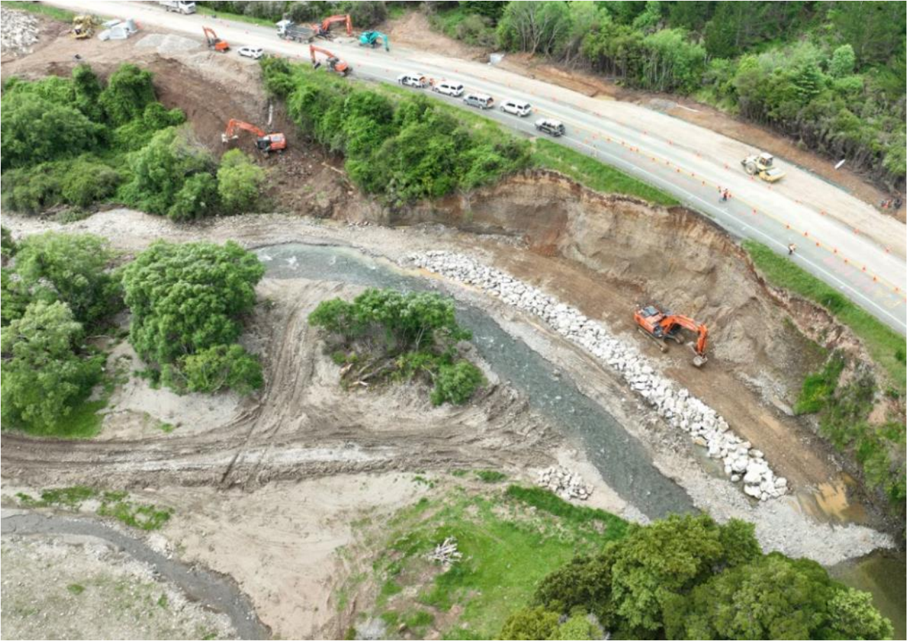
Figure 2: - works being undertaken during SH6 road closure
