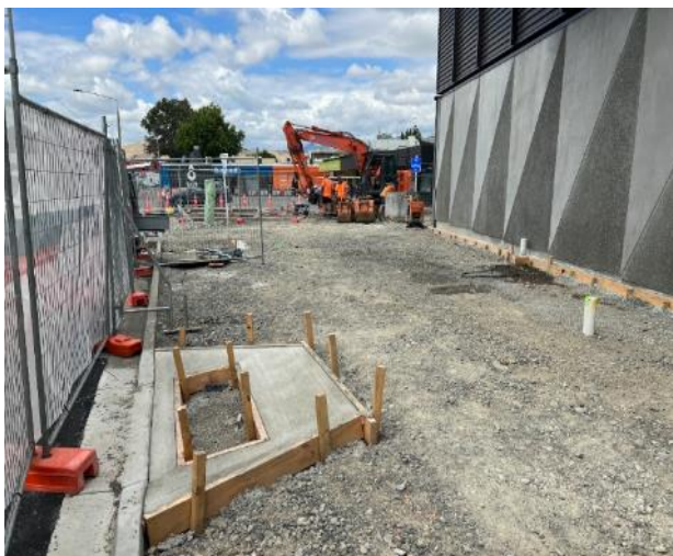
Fig 7 – Symons St, Blenheim Streetscape Upgrade
