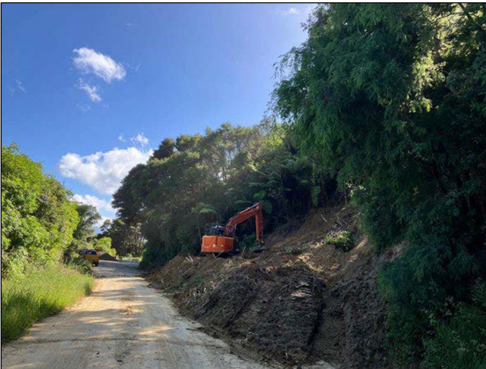
Crews working on Kenepuru Road near Tara Bay Road
