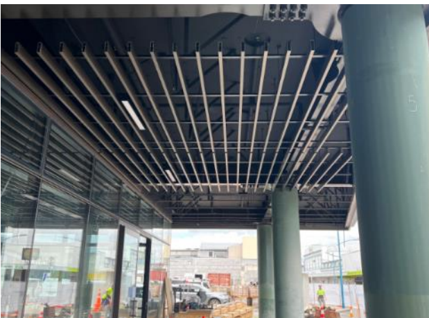
Fig 13 – Decorative timber cladding - MLAG
