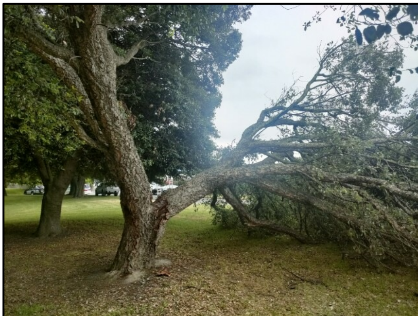
Tree removal probably required after substantial branch loss from Cork Oak on Murphy's Creek Reserve
