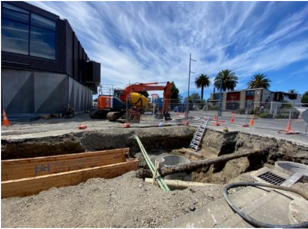
Fig 9 – Storm water upgrade, Blenheim Streetscape
