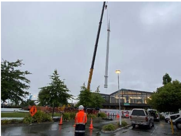
Fig 1 – Echo Mast installation, The Quays
