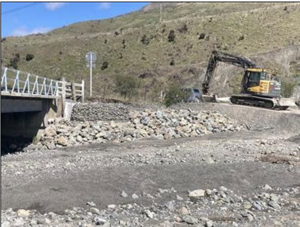
Scour repair at Castle Bridge in Awatere Valley
