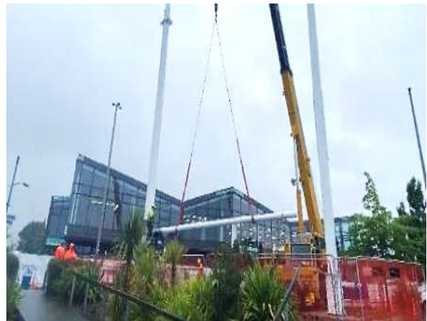
Fig 2 – Echo Mast boom installation, The Quays
