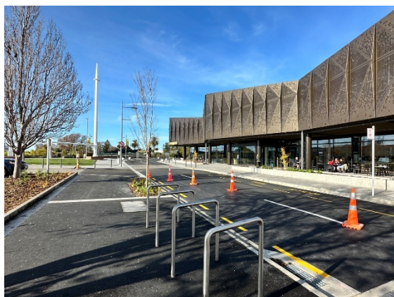
Fig 3: Streetscape upgrade, High Street
