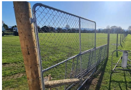
Fig 16: Hockey Turf project, site fencing installed and awaiting scrim
