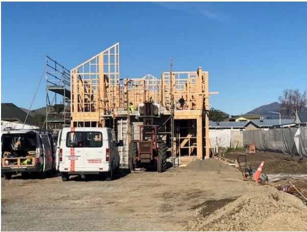
Fig 11: 85 George Street development, second storey framing going up
