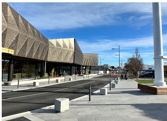
Fig 2: Streetscape upgrade, MLAG
