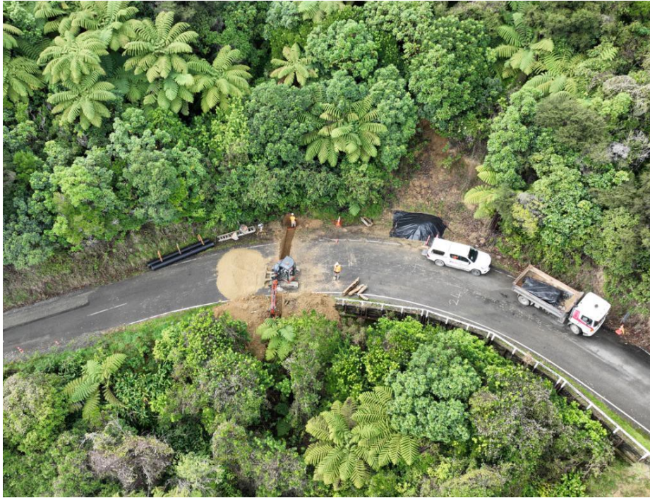
RJ Civil undertaking culvert replacements on Kenepuru Road – image taken 30 May 2023
