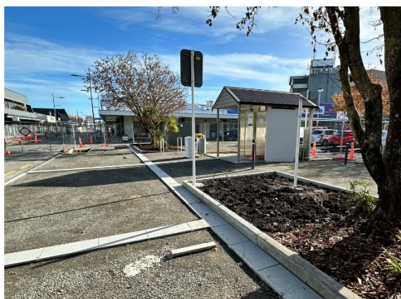
Fig 4: Streetscape upgrade, High Street toilet
