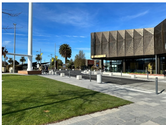
Fig 1: Streetscape upgrade, The Quays
