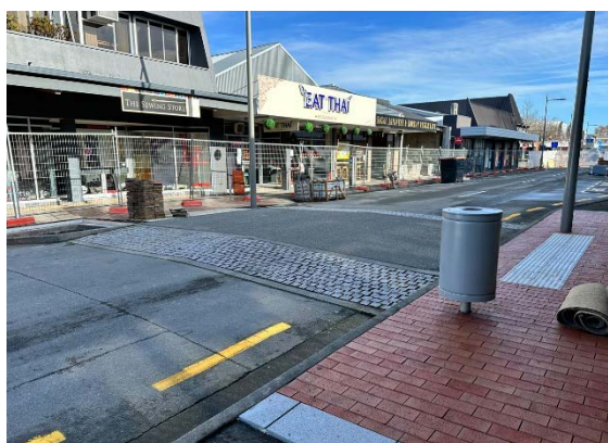
Fig 5: Streetscape upgrade, High Street west
