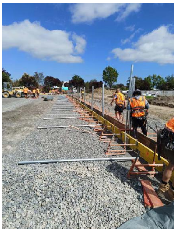
Figure 4 – Hockey Turf concrete nib, Nelson
