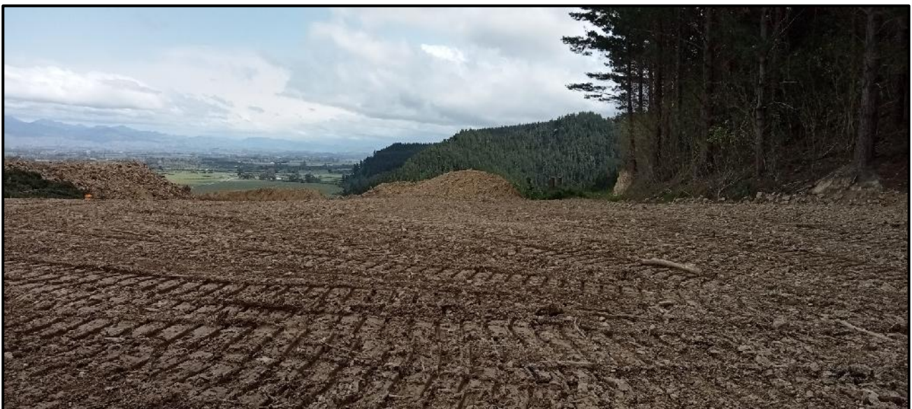
Figure 2 – back boundary topsoiled ready for grassing and fencing
