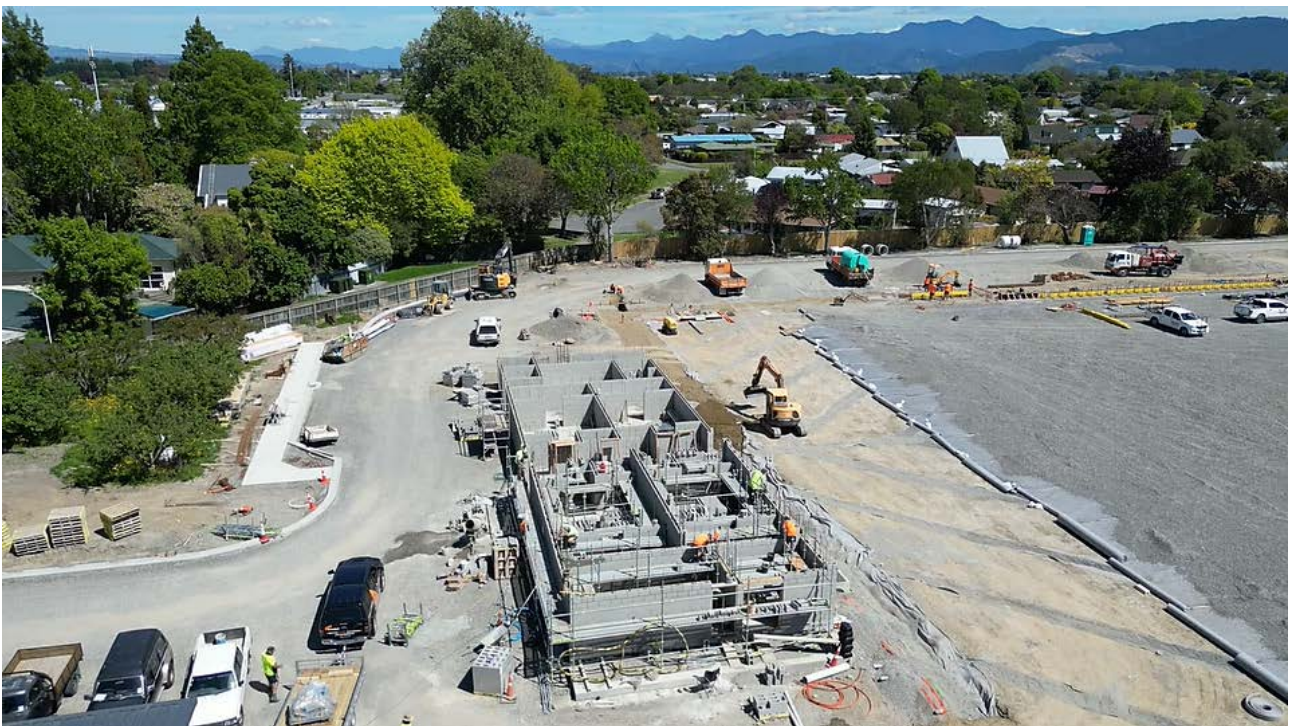
Figure 7 – Hockey Pavilion, Nelson Street
