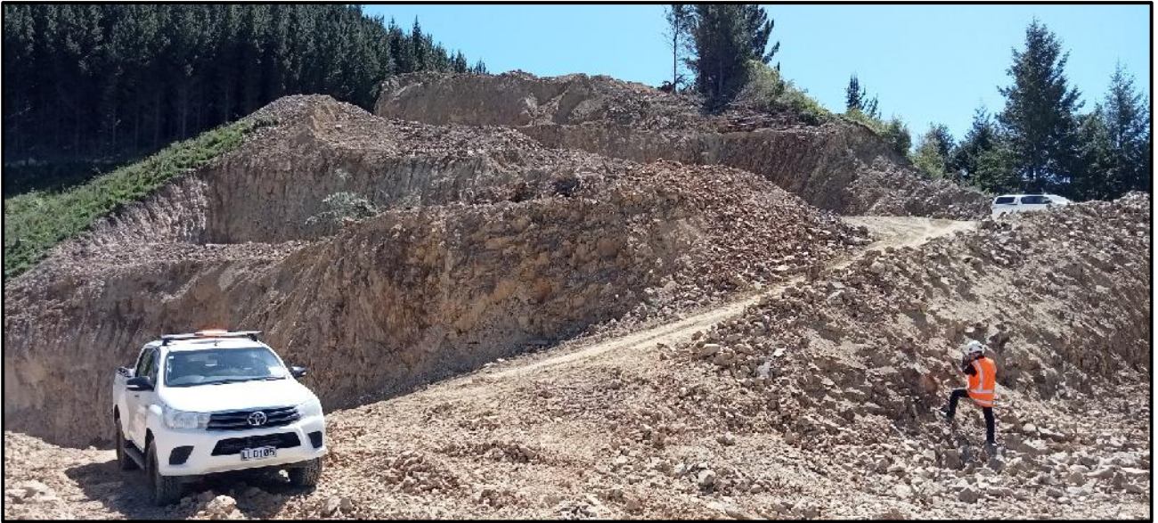
Figure 3 – benching main face
