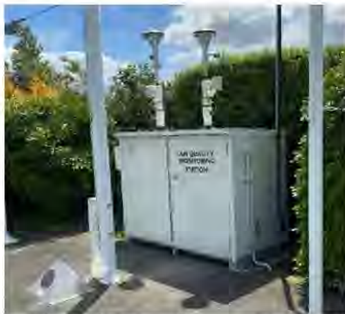
Photo 1 – Air quality PM monitoring site in Blenheim
