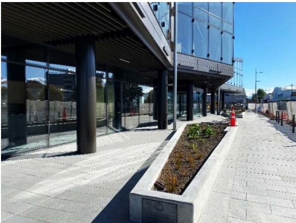
Fig 7: Streetscape upgrade, paving laid.
