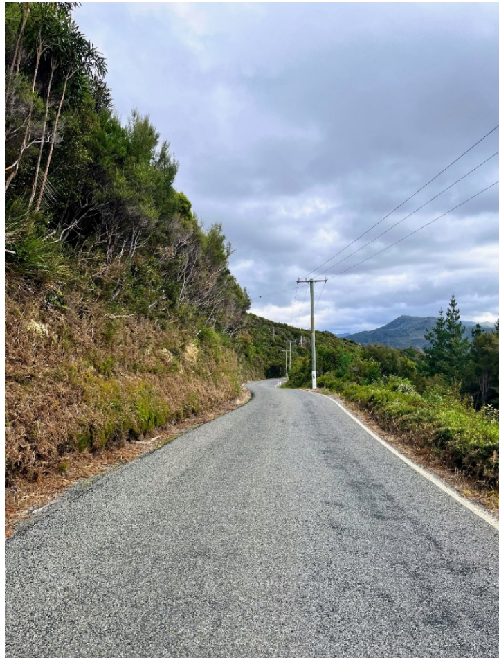
Fig. 18 -Vegetation has been trimmed on French Pass Road to maintain sight lines
