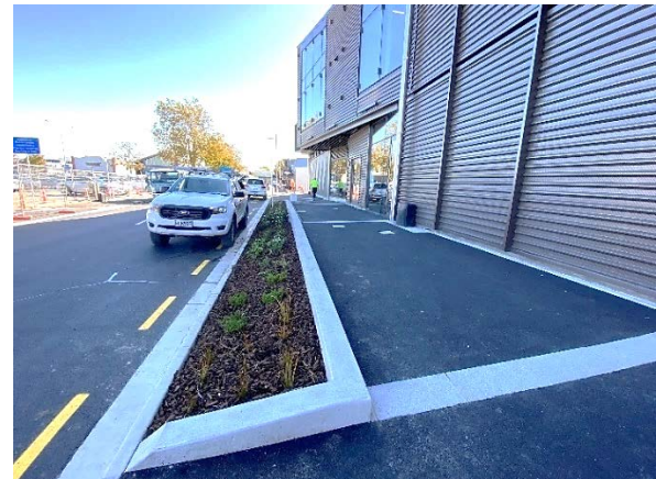
Fig 8: Streetscape upgrade, Wynen St complete
