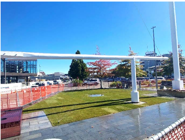
Fig 3: Turf reinstated at The Quays
