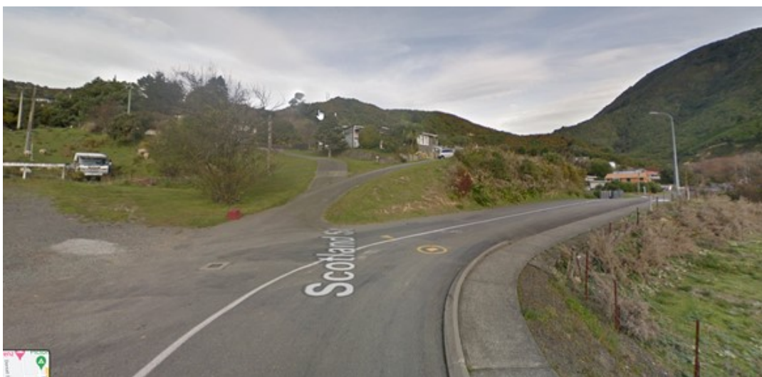
Fig. 19 – Scotland Street example of an area of unformed road
