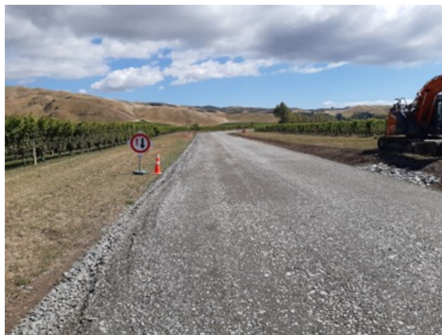
Fig. 8 – 17 February completion of works prior to harvest
