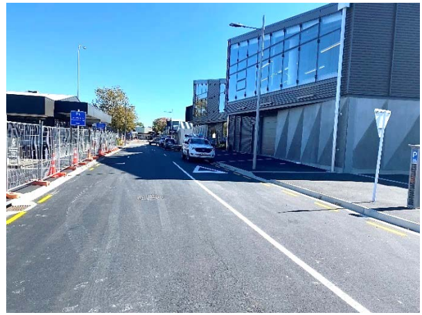
Fig 10: Wynen Street newly asphalted
