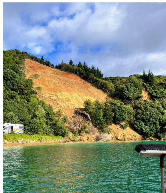
Fig. 14 – Repaired slip at Elmslie Bay
