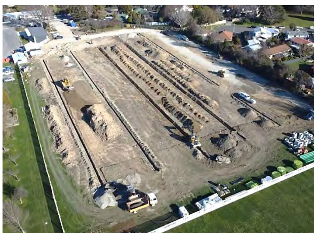
Figure 1: Hockey Turf – Excavation underway
