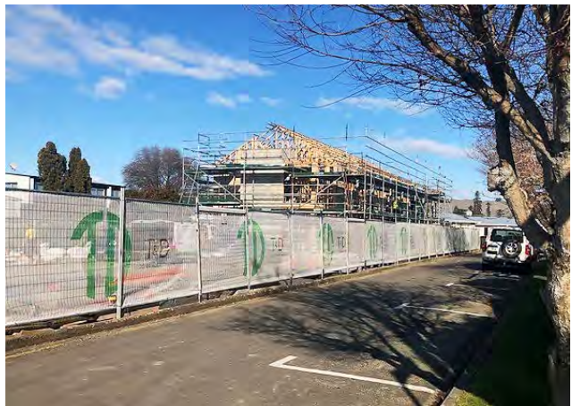
Figure 12: 85 George Street, Senior Housing development
