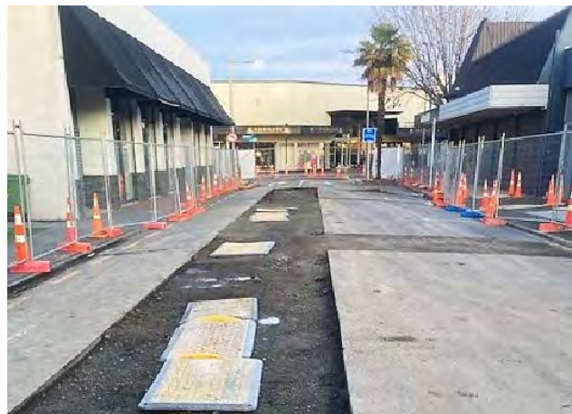
Figure 6: Blenheim Streetscape - Storm water renewal trenching filled on Wynen Street
