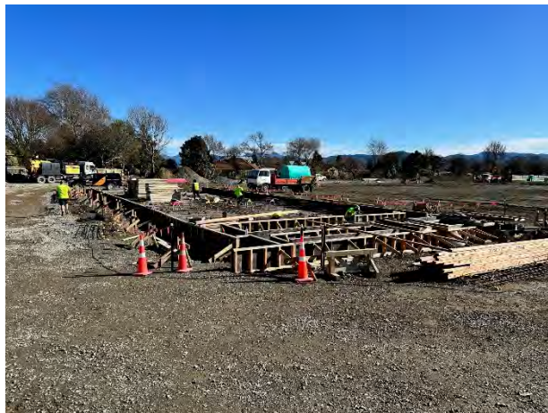
Figure 4: Hockey Pavilion – Boxing foundations
