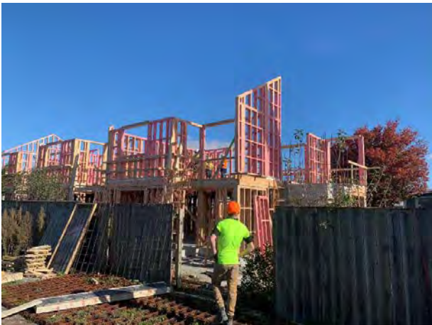
Figure 11: 85 George Street, Senior Housing development
