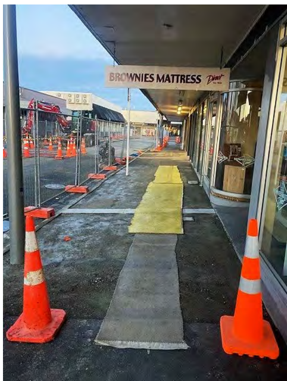
Figure 7: Blenheim Streetscape – Footpaths ready for asphalt in mid-August
