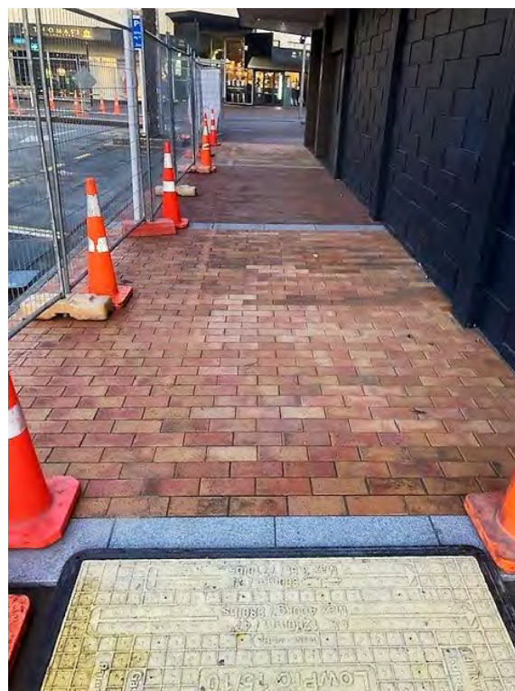
Figure 8: Blenheim Streetscape – New (non-slip) clay brick paving laid outside Michael Hill on Wynen Street
