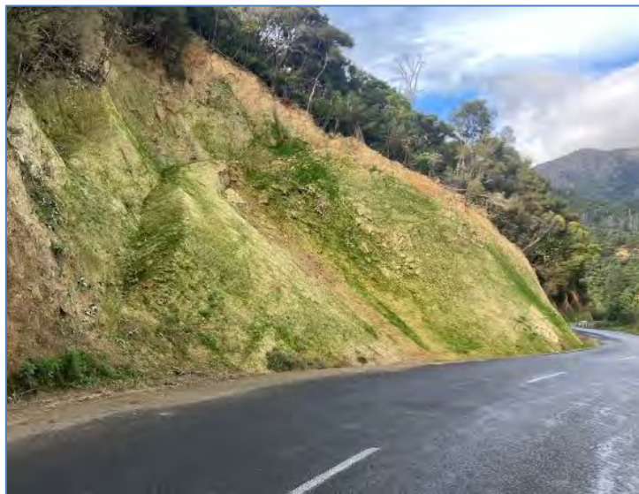
Vegetation beginning to take hold along Queen Charlotte Drive – image taken 20 July 2023
