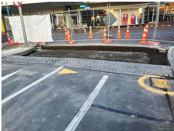
Figure 5: Blenheim Streetscape - Renewed pedestrian crossing on Cnr Market and Wynen
