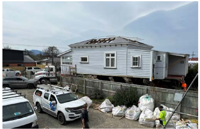
Figure 18 – 83 George Street, house removal
