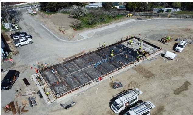
Figure 1 – Hockey Pavilion, Nelson Street
