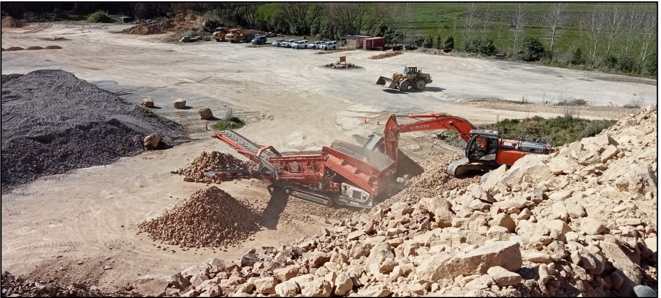
Figure 3 - screening of rubble products for planned early 2024 Wairau Diversion repairs
