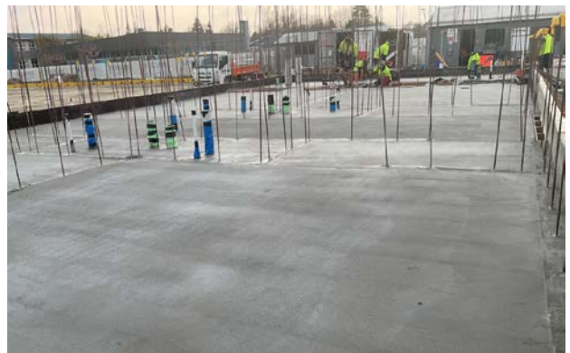
Figure 6 – Hockey Pavilion slab, Nelson Street
