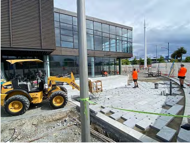
Fig 5 – Streetscape Upgrade – paving underway
