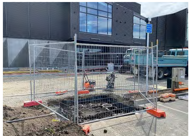
Fig 10 - Streetscape Upgrade, pits for new street trees
