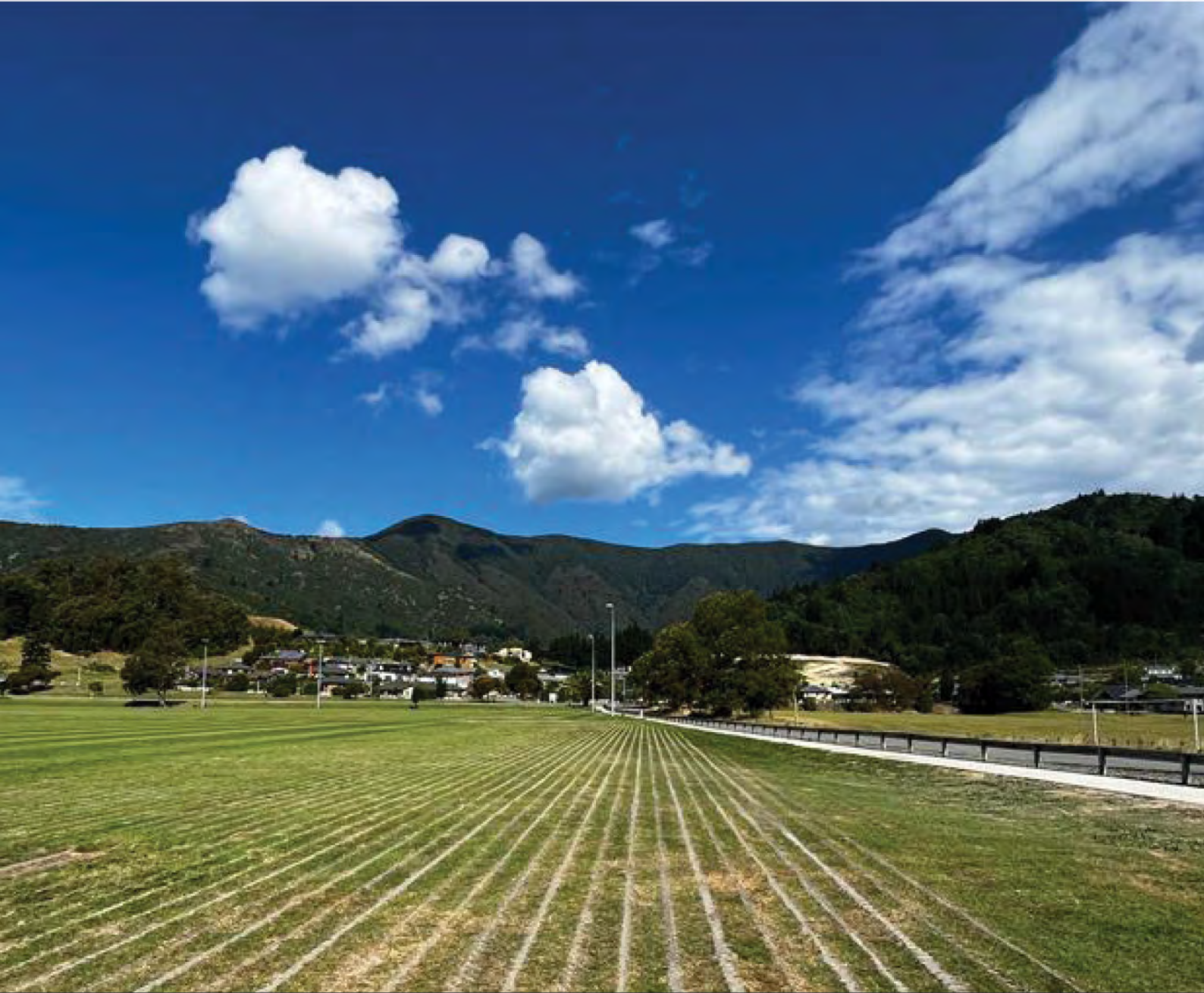
Endeavour Park, Picton - Gravel banding on playing surface
