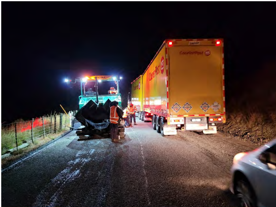
Figure 2 – Welds Pass Maintenance
