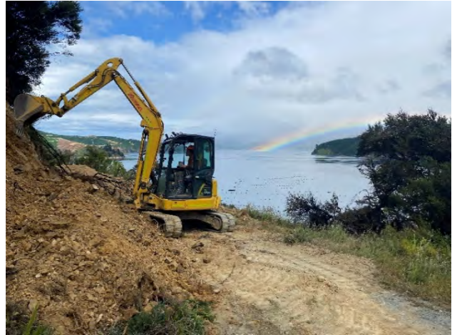
Noel Bridge construction
