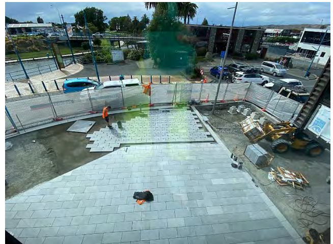
Fig 8 - Streetscape Upgrade, paving underway
