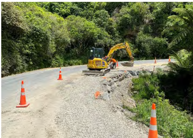
Improved access in progress on Kenepuru
