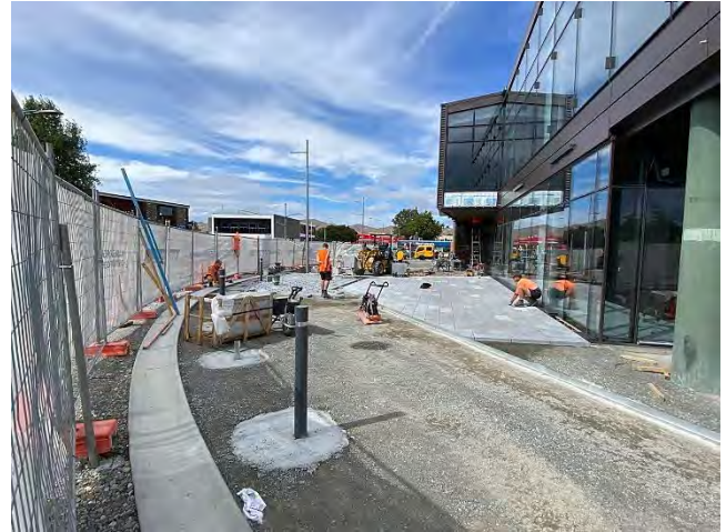
Fig 6 - Streetscape Upgrade, paving underway
