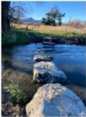
Figure 7 - Wairau River - Installed stepping stones
