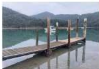
Figure 11 - Completed Repairs - Duncan Bay Jetty
