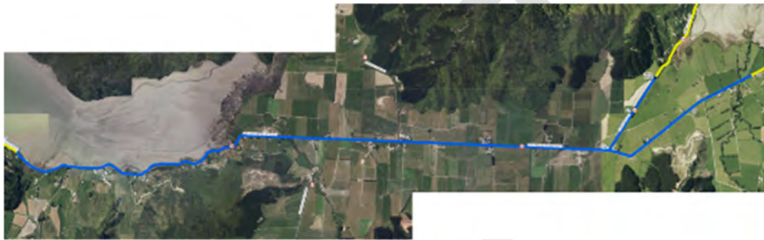
Figure 32 Grove Track - Linkwater
