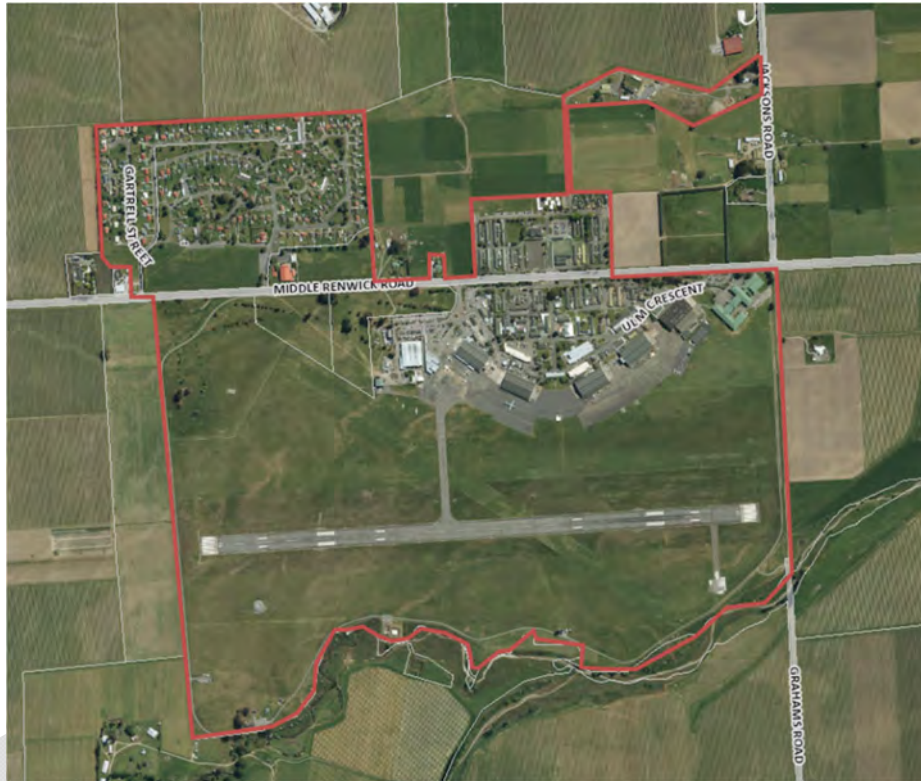
Figure 6 Ministry of Defence Roads
