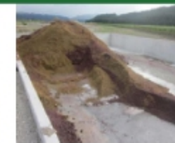
Sealed storage area with leachate collection
