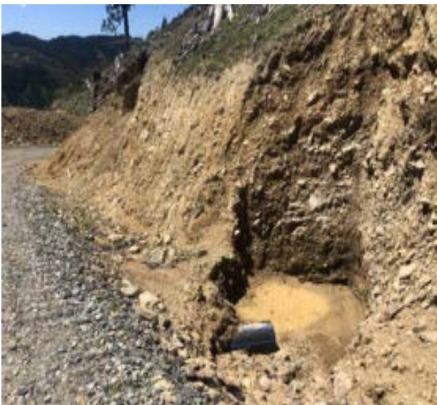
Figure 4: Full Sediment controls.
