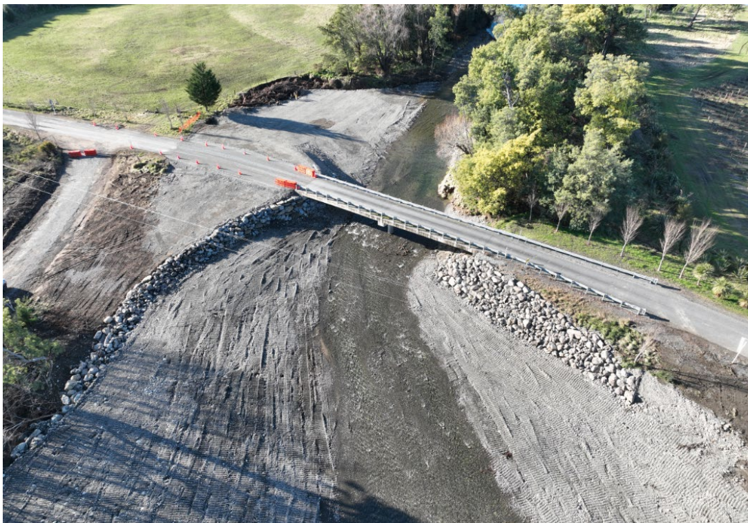
Figure 9 - Approach Reinstated at Tyntesfield Bridge
