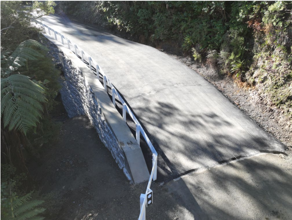
Figure 3- Completed Retaining Wall Tennyson Hill
