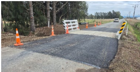
New bridge deck - Hardings Road
