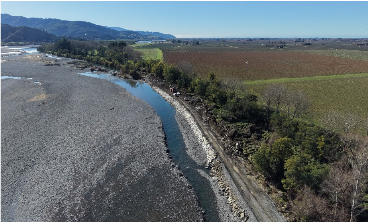
Giffords Road project progress 28/07/26
