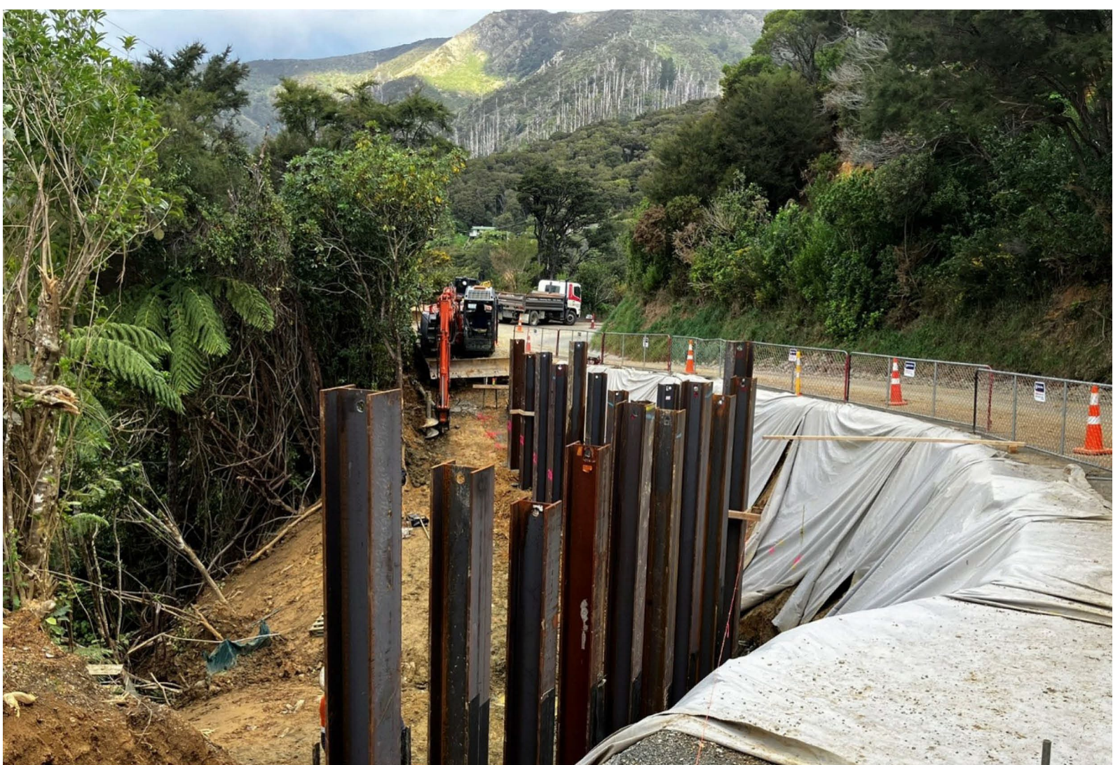
Retaining wall under construction Queen Charlotte Drive
