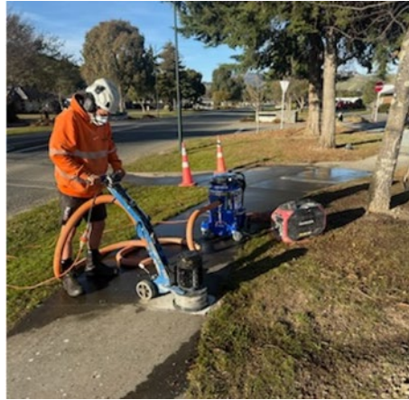
Taylor Pass Road footpath repairs
