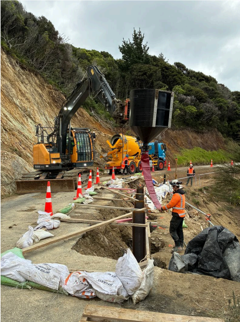
Figure 2- Concreting Piles French Pass
