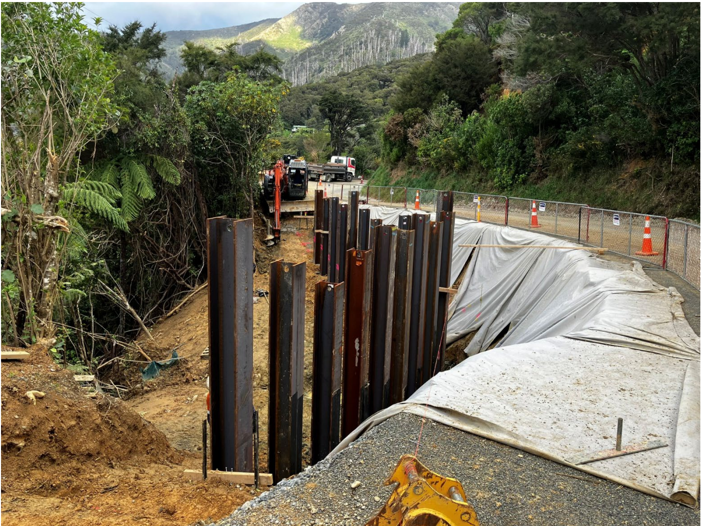
Figure 6-Retaining Wall under Construction Q C Drive
