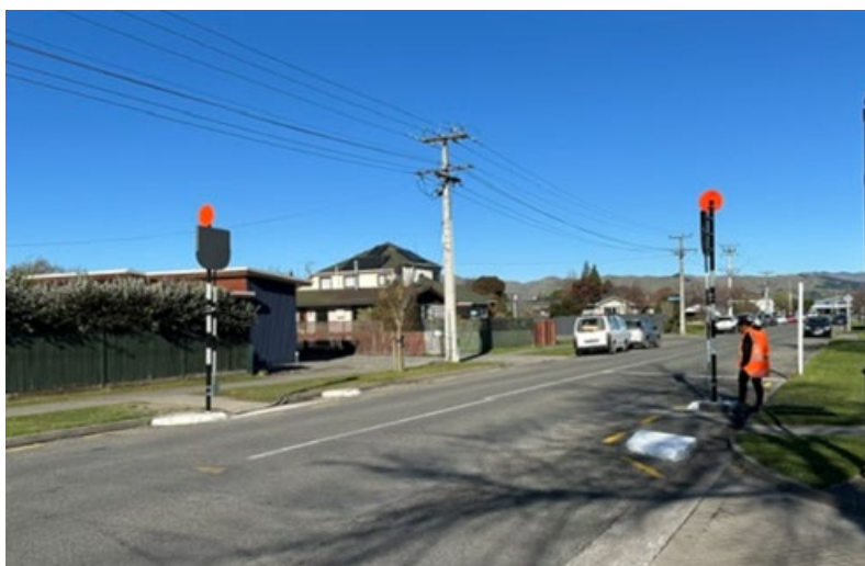
New Kea Crossing on Hutchinson Street
