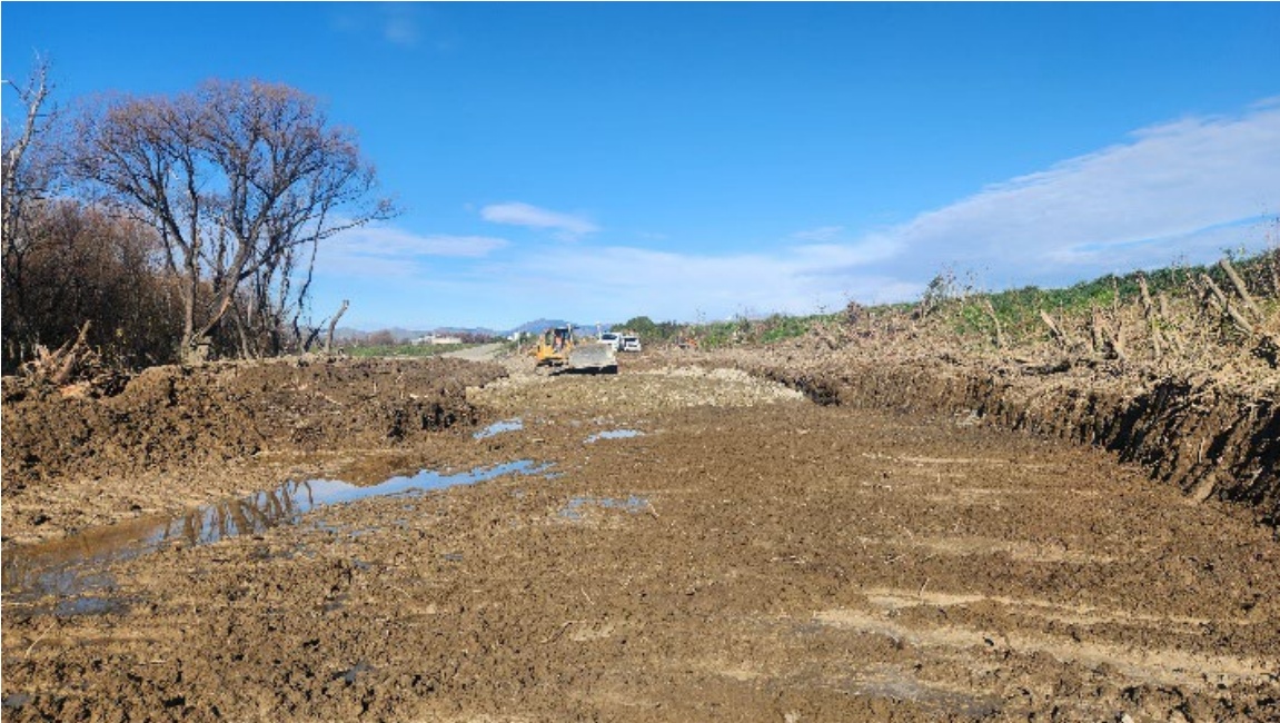
Upper section : no-rip rap reach
