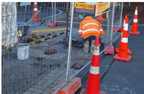
Seventh Lane repair works
