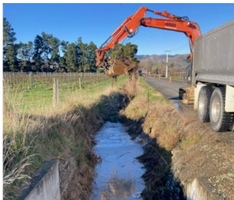
Ben Morvan Road water channel clearance works
