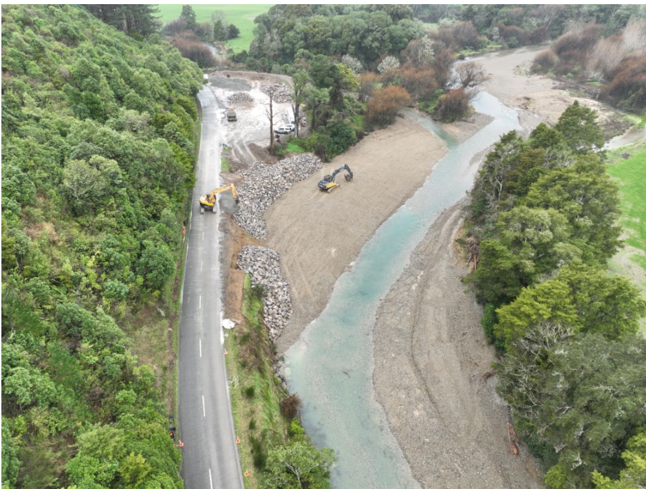
Figure 1-Rock protection works Ronga Road
