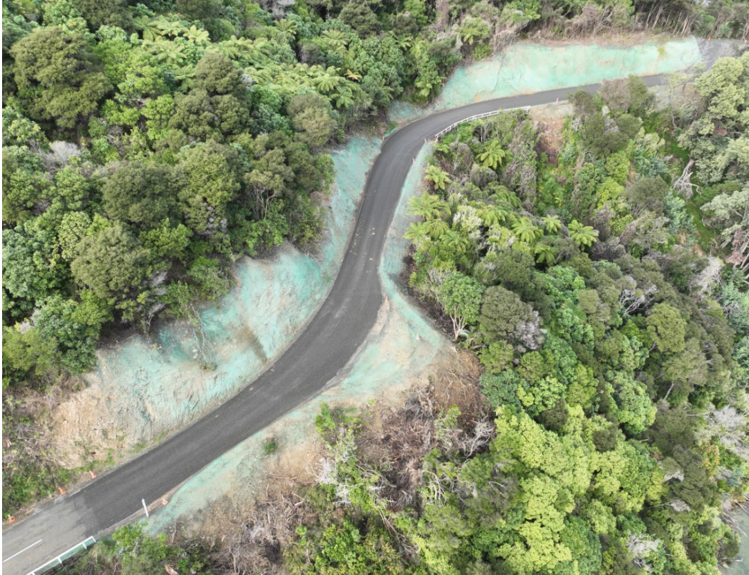
Figure 4- Completed Road Retreat Kenepuru Road
