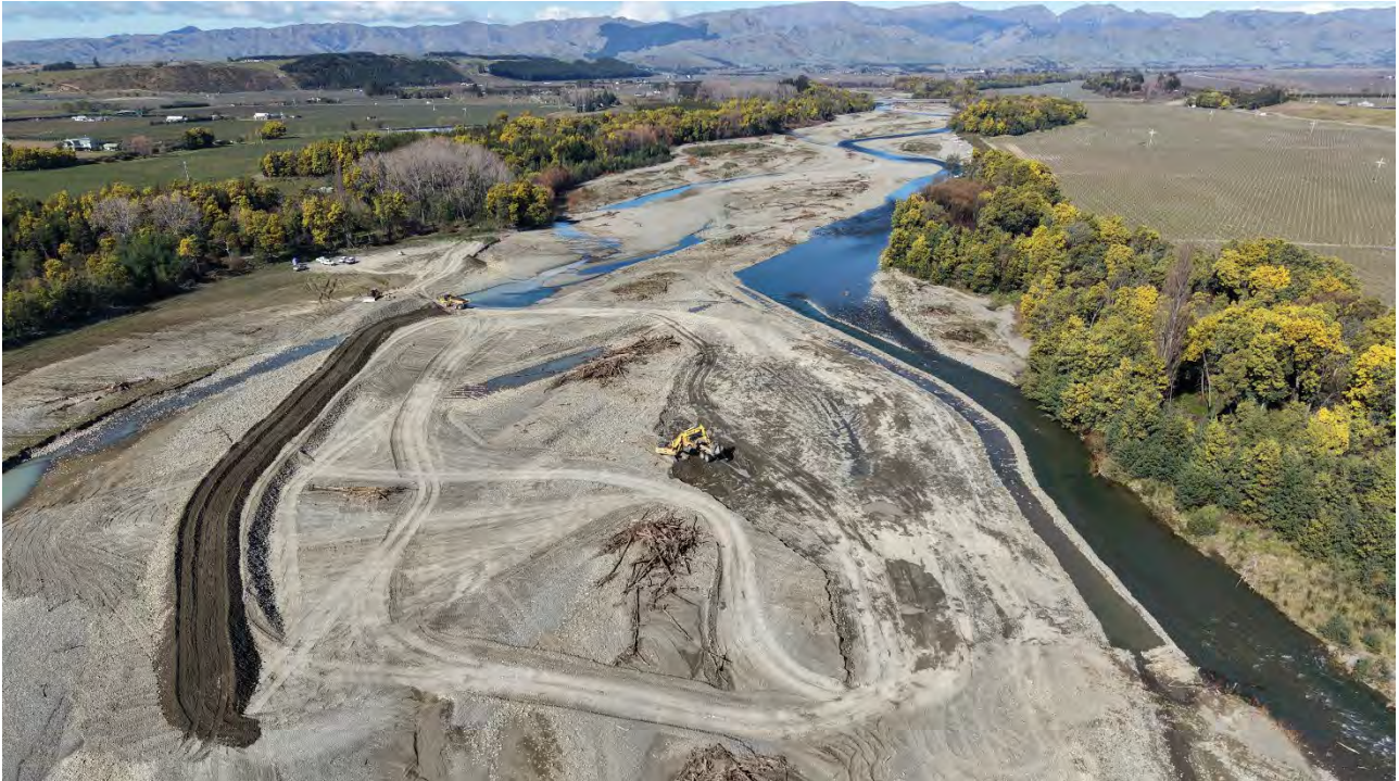
Figure 7: Looking upstream. Temporary repair works nearing completion in July 2026, including river realignment and reinstatement of the gravel bund for stopbank protection.
