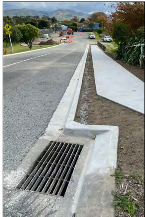
Figure 8 Newcome Street Seddon - New footpath from corner of SH1
