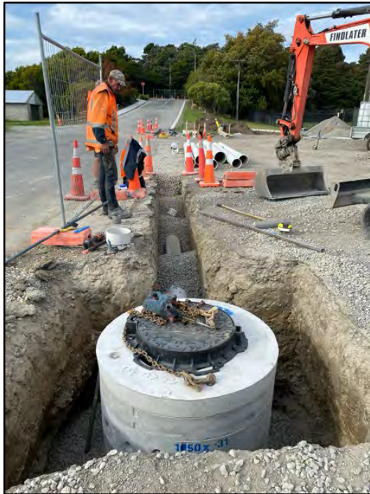
Figure 5 Newcome Street Seddon – Stormwater infrastructure being installed
