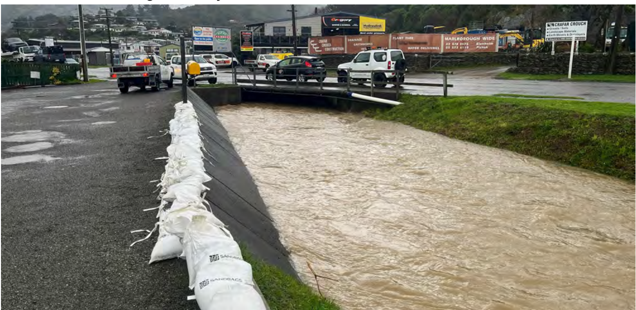
Figure 14: Kent Street Drain below Dublin Street a few hours after the peak flow in July 2026
