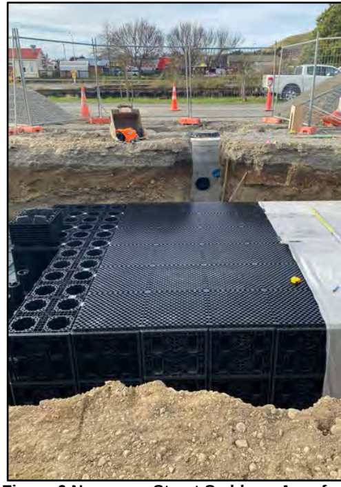
Figure 6 Newcome Street Seddon - Aquafort Soakpit being installed
