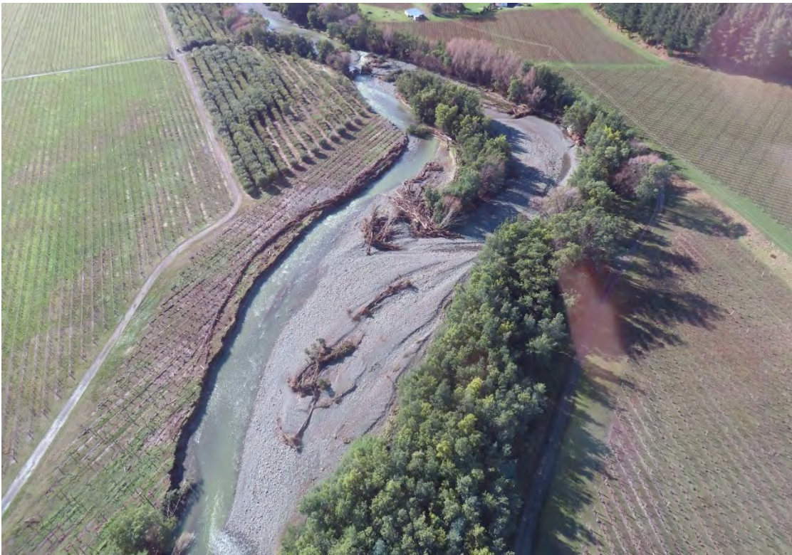
Figure 16: Omaka River between Lake Timara Ford and Tyntesfield road bridge, river escaped existing channel during July 2026 event
