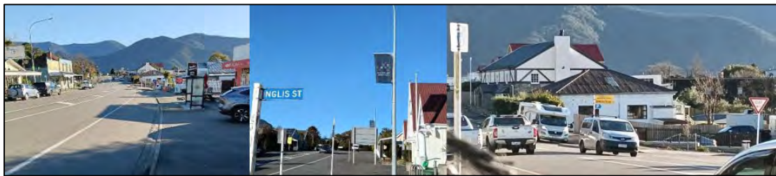
Figure 1 State Highway 6 Main Street Havelock - looking north and south
