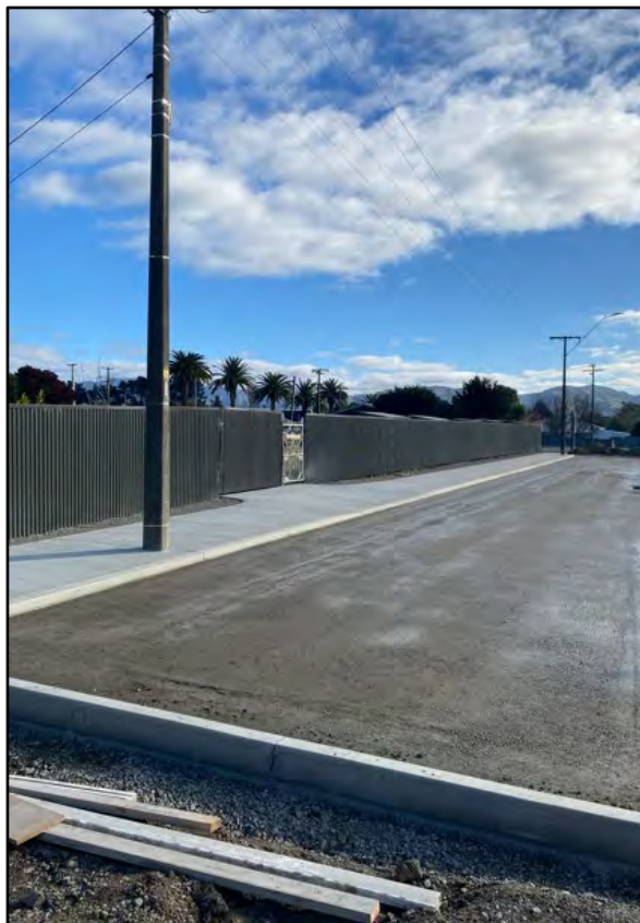
Figure 7 Newcome Street Seddon - new footpath adjacent to Bowling Green and carpark prepped for sealing
