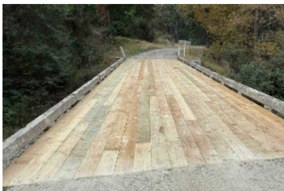
Deck Repairs at Enchanted Bridge, Northbank
