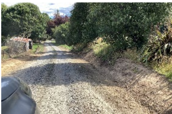
High Shoulder works at Peakes Road
