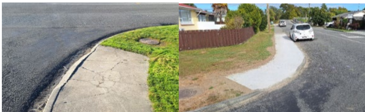
Example of footpath before and after repair work
