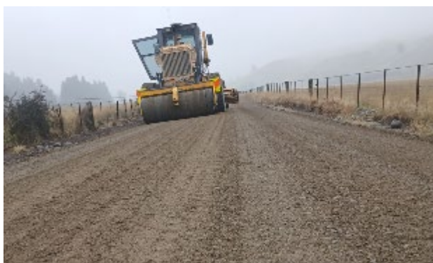
Resheeting works at Avon Valley Road
