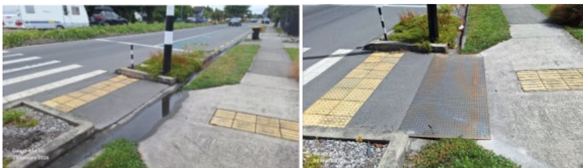
Nelson Street crossing before and after works
