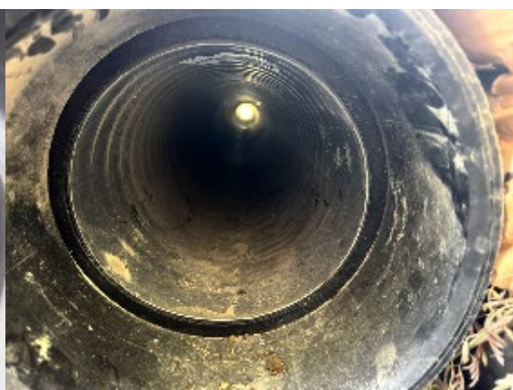
Culvert on Croisilles Road after works
