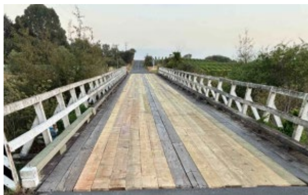
Deck Repairs at Brancott Road No.2
