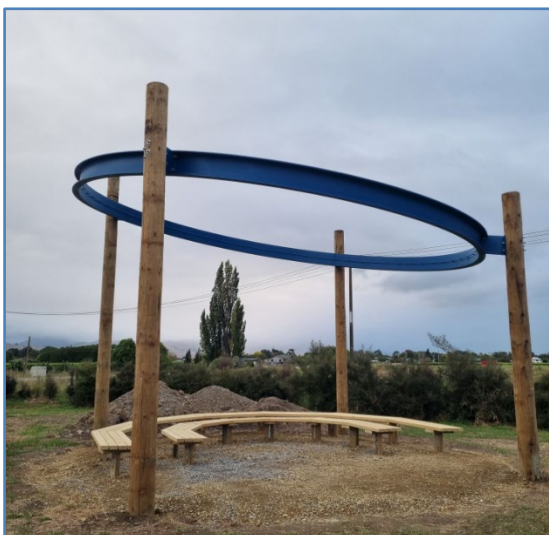
Figure 2 Grovetown - work in progress on the new Kura gathering space
