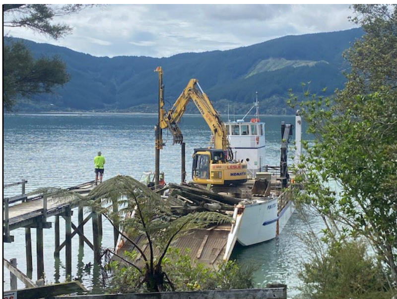
Figure 5 Whatanihi Jetty - work underway
