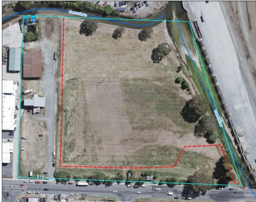
Figure 1- 2015 Aerial – Former Rugby Pavilion and Sports Centre (Squash Building)
