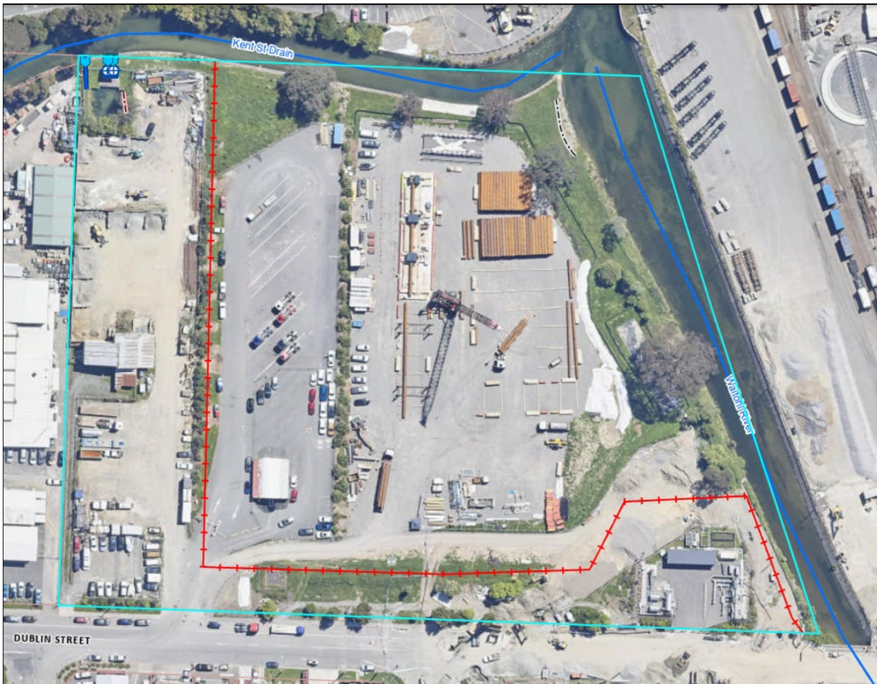
Figure 3 – 2023 Aerial displaying area being used for I-Rex staging
