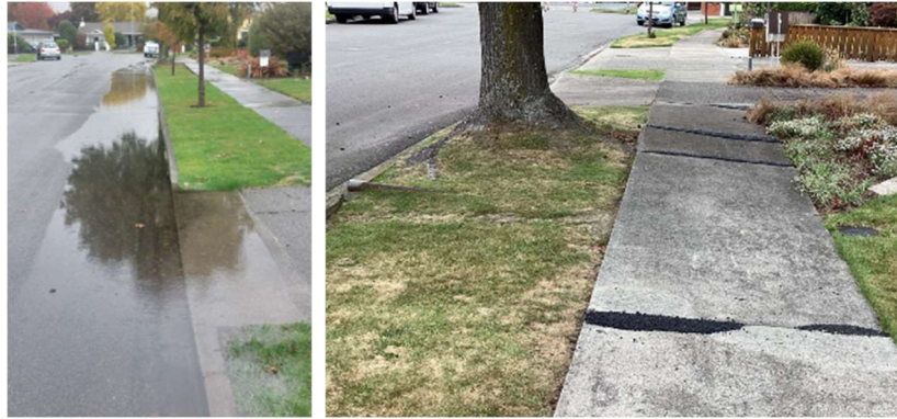
Manor Place – footpath repairs
