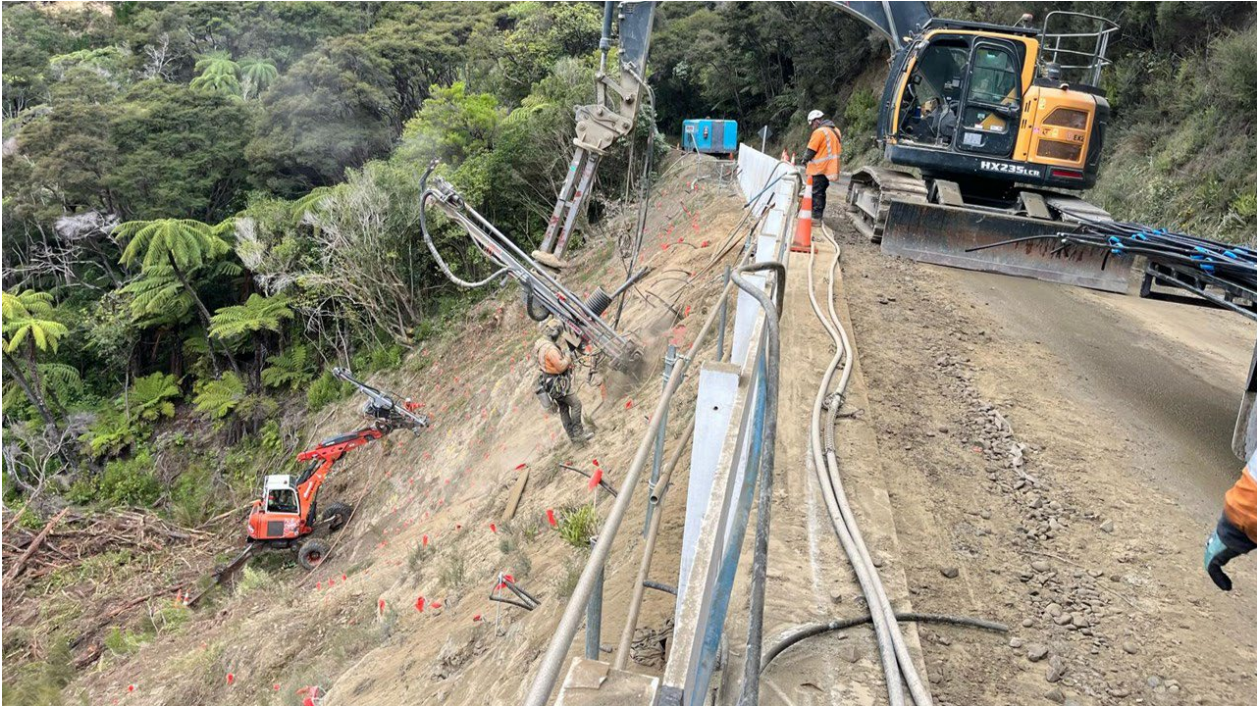
Figure 1- Drilling Anchors Kenepuru Road
