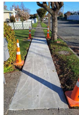
Glover Crescent – tree root damage repairs
