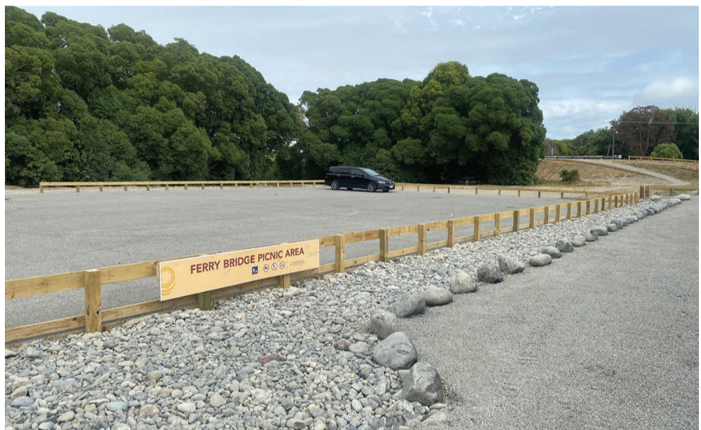
The revamped Ferry Bridge carpark
