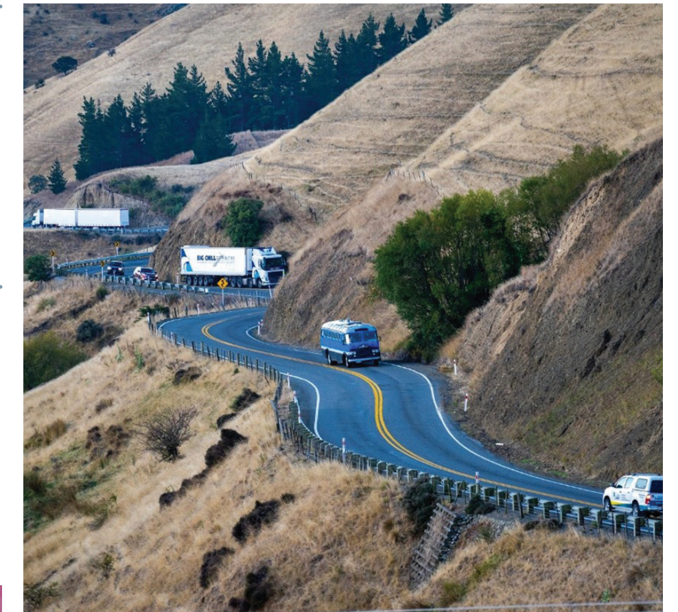
Weld Pass is to close during February
