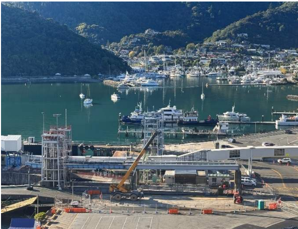
Contractors on site at Port Marlborough preparing to de-construct the remainder of the Vehicle Access Bridge and linkspan
