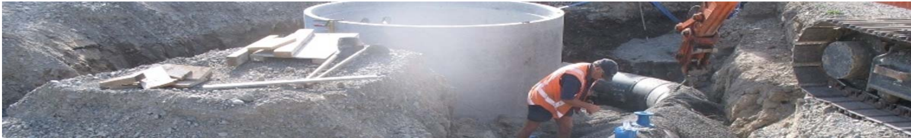
Photo: Construction of the Central WTP Reservoir, Blenheim
