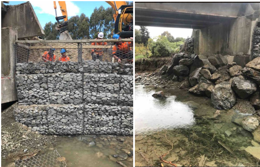
Structural Repair work at the Enchanted Bridge site
