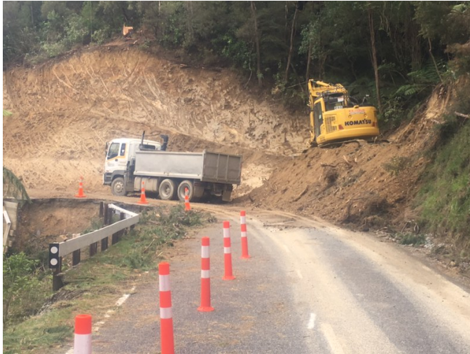
Slip clearance on Kenepuru Road - between Linkwater and Mahau Road
