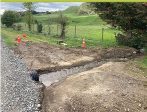
A blocked and damaged 300mm culvert at 11.8km was replaced with a 450mm culvert
