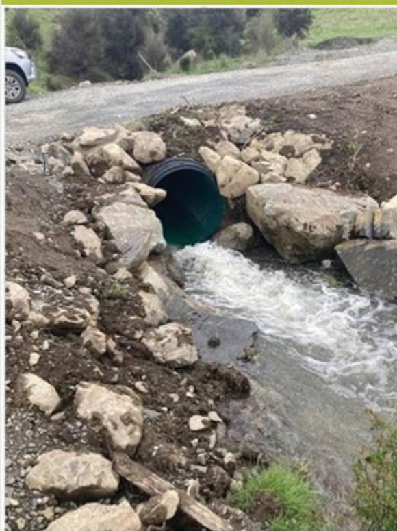
Rock armouring at the inlet and outlet of a 900mm culvert at 6.7km
