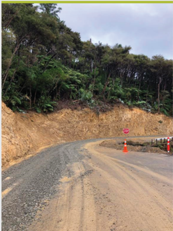
Approximately 3,000 cubic metres of material has been removed from these slips
