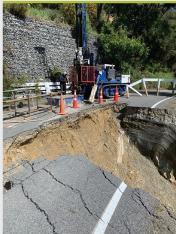
Drill Rig working at slip site 28.5km from Linkwater
