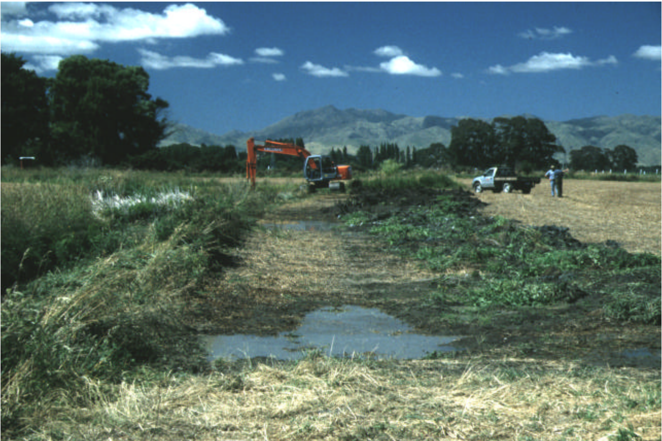
Figure 4.1 Mechanical clearance of Giffords Creek December 1999.
