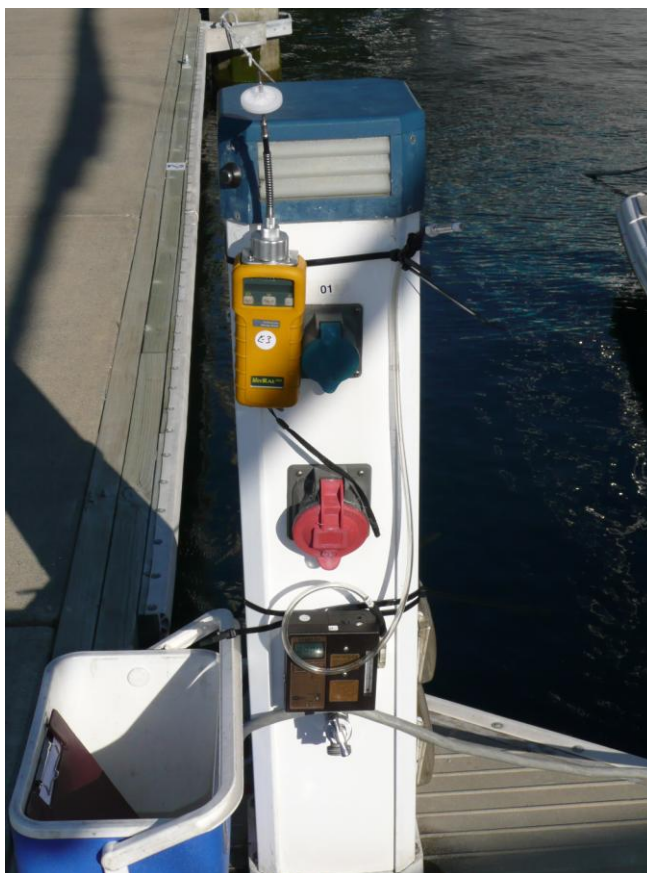
■ Figure 4: Picton Jetty PID Monitoring Site
