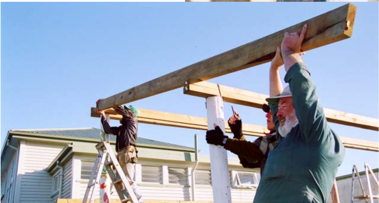
Raising the rafters; Steve Dowell helps Murray Ward lift a support beam into place.
