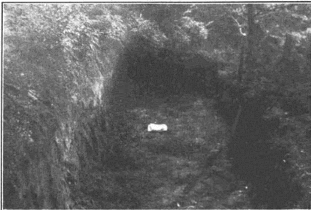
Figure 3-1: An old pit dwelling (top) from McIntosh et al. (1940), and (below) another from Elvy (1926).
