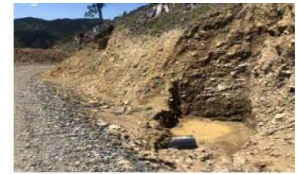
Full sediment controls
