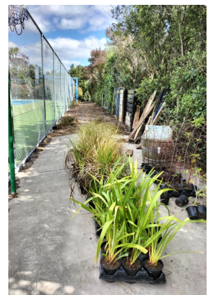
After and ready for planting
