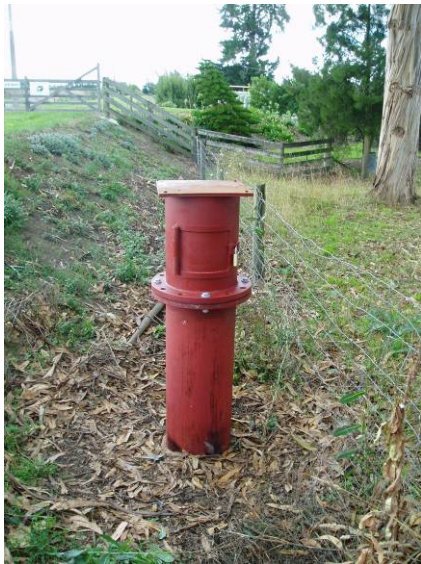
Figure 31 : Well P28w/4404 looking west with Opawa River in background by willow trees
