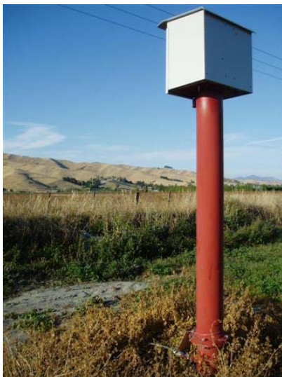
Figure 51 : MDC permanent monitoring well 4402 looking south-west towards Wither Hills
