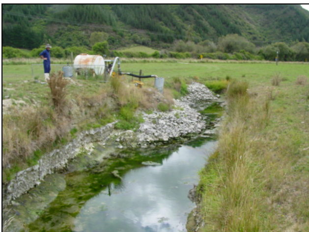
#26 P27w/0496 Delany irrigation pit
