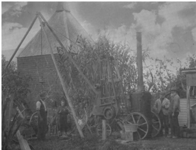
Figure 3.17: Thomas Cragg and Sons operating a steam powered cable tool rig at Grovetown Hotel around 1900 (Marlborough Historical Society)
