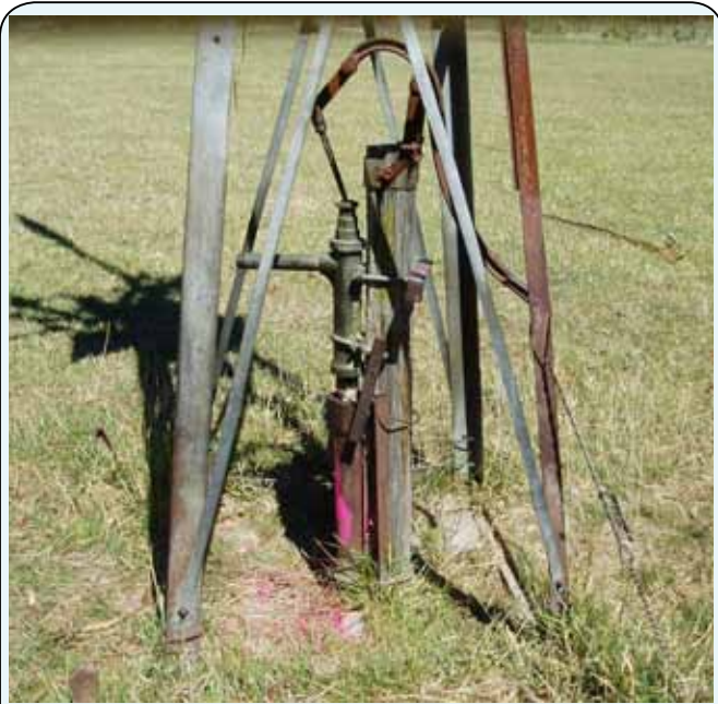
Figure 3.27: Close-up of well at Shep's Park Reserve. Groundwater flows out of the horizontal pipe as the curved handle is moved up and down by the turning of the wind vanes.
