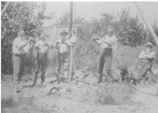
Figure 3.16: Thomas Cragg and Sons using hand operated well drilling equipment about 1900 (Marlborough Historical Society)
