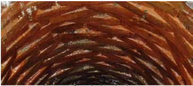
Figure 3.5: Close-up of interlocking bricks
