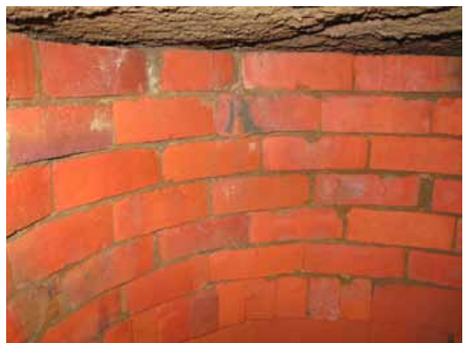
Figure 3.23: Cemented brick lined well
