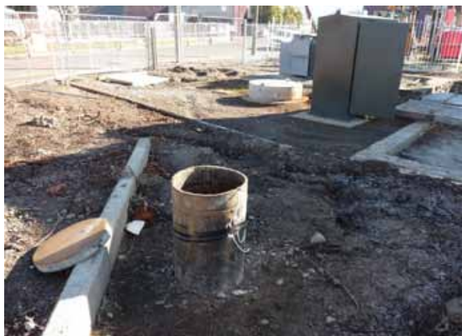
Figure 3.25: Upgrading and redevelopment of Grove Road municipal wellfield 2010
