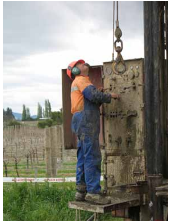
Figure 3.30: John Butt constructing MDC Spring Creek effluent treatment pond well
