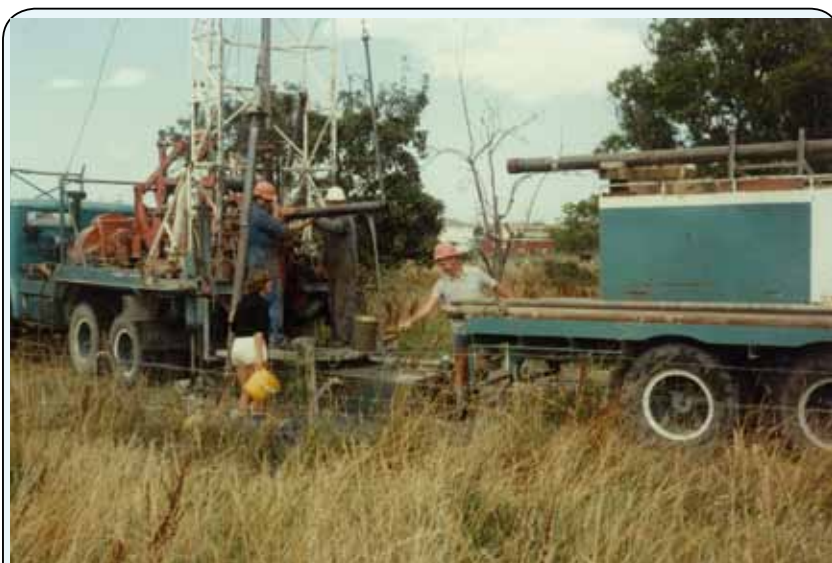
Figure 4.3: Len Brown of the NZ Geological Survey logging the drill cuttings as they arrive at the surface during the drilling of a Kaikoura well in the 1980s. He is holding a sieve to collect the material for inspection and recording.
