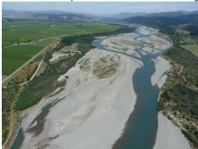
Figure 17.25: Wairau River recharge reach
