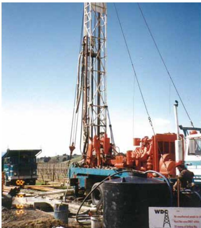
Figure 30.2: Exploratory well 2917 under construction
